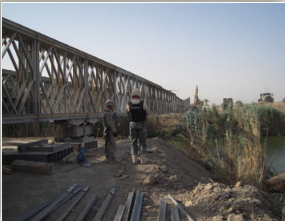
Staff Sgt. Floyd Hathaway, 401st EN CO, build commander, along with a Mabey Bridge & Shore Inc. representative overlook the 16-bay, 160 feet long span on the Hamadi Bridge in May of 2009. (Photo courtesy of Staff Sgt. Floyd Hathaway)
