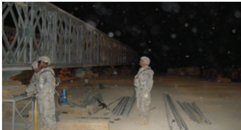
Members of the 401 EN CO steady work into the night on the longest single span Mabey Johnson logistic support bridge in Iraq. (Photo courtesy of Staff Sgt. Floyd Hathaway)
