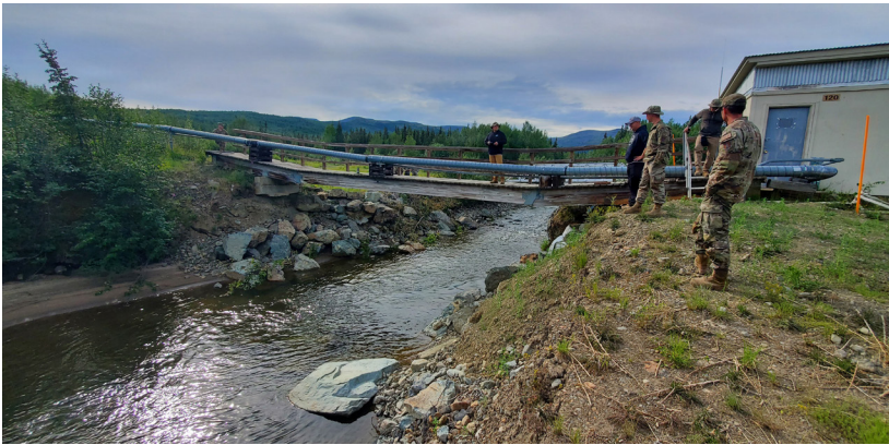
Airmen from the 173rd Fighter Wing's Civil Engineering Squadron repaired the sole water line during Operation 26-02 Indian Mountain at Indian Mountain Long Range Radar Station in Alaska on July 9, 2026. Fixing the bridge ensured proper sanitation and fire suppression for the nearby facility. (Courtesy photo, 173rd CES)
