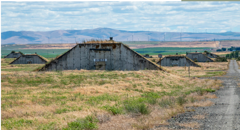
Rows of 'igloos' at the former Umatilla Chemical Depot once stored military ordnance and chemical weapons while the site was active. At its peak, the depot held about 12 percent of the U.S. chemical weapons stockpile. These bunkers are 80 feet long and 30 feet wide, fitted with a 5-foot-by-10-foot steel doors.
