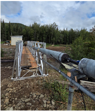
The rebuilt bridge completed by 173rd CES members at at Indian Mountain Long Range Radar Station, in Alaska. (Courtesy photo, 173rd FW CES)
