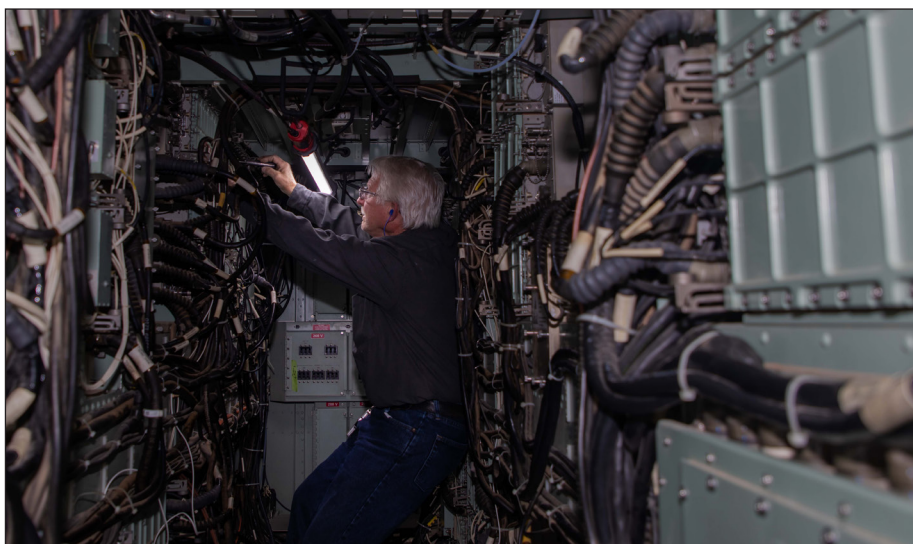
Jeffrey Traini, a Letterkenny Army Depot electronics mechanic, straps cables on a Patriot RADAR at Letterkenny Army Depot, June 1, 2021. This insider's view of integration shows an example of the additional layer of complexity that cable routing and component layering adds. LEAD's engineering services framework helps to demystify the troubleshooting and repair process by providing warfighters and depot subject matter experts with a common operating picture of the delivered asset.
