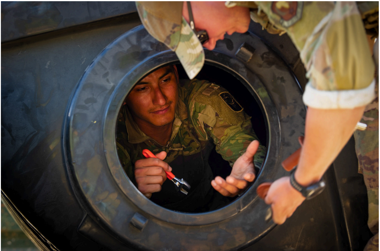
U.S. Army SGT Leonardo Garcia, assigned to Combat Company, Task Force Seminole, installs a water tank at Manda Bay, Kenya, Aug. 12, 2026. (U.S. Army photo by SGT Jake Anico).
