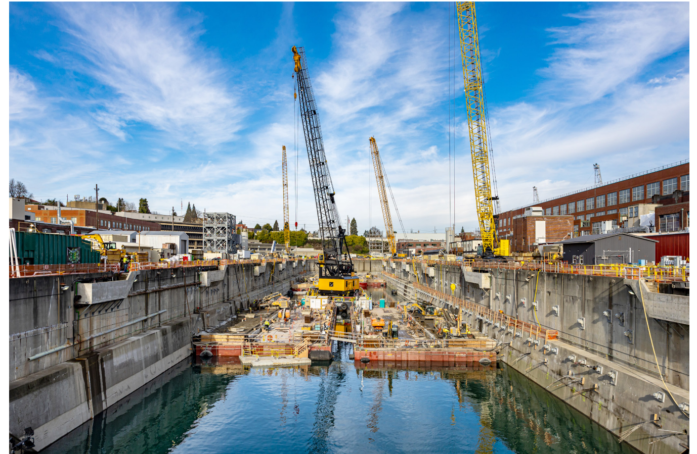
ABOVE: Seismic retrofit work on Dry Dock 4 at PSNS & IMF was completed on budget and ahead of schedule, thanks to crew members who worked around the clock, six days a week to finish the modernization project. (U.S. Navy photo by Jeb Fach)
