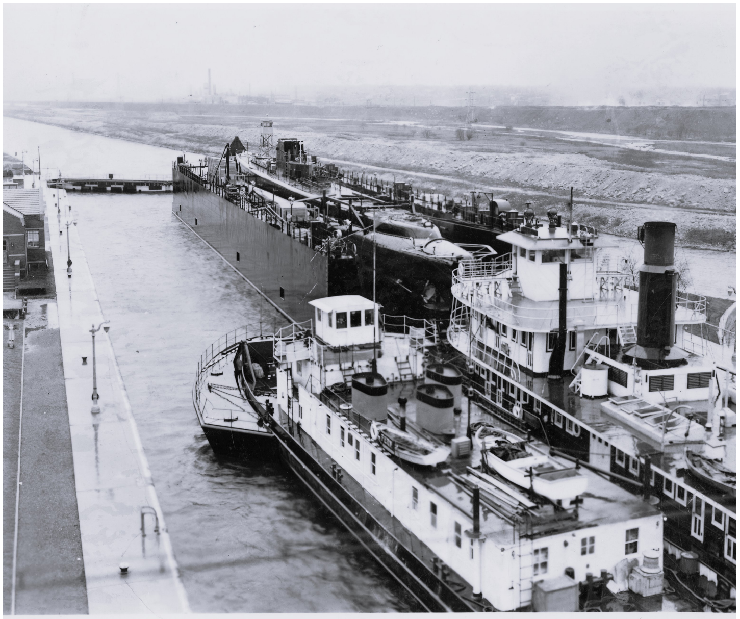
Looking down from Lockport Lock's lift tower in 1942, the submarine USS Peto traverses the Illinois Waterway in a floating drydock. Whether moving emergency wartime vessels or millions of tons of agricultural and industrial goods each year, U.S. Army Corps of Engineers navigation infrastructure has been vital to the process. District Library Photo
