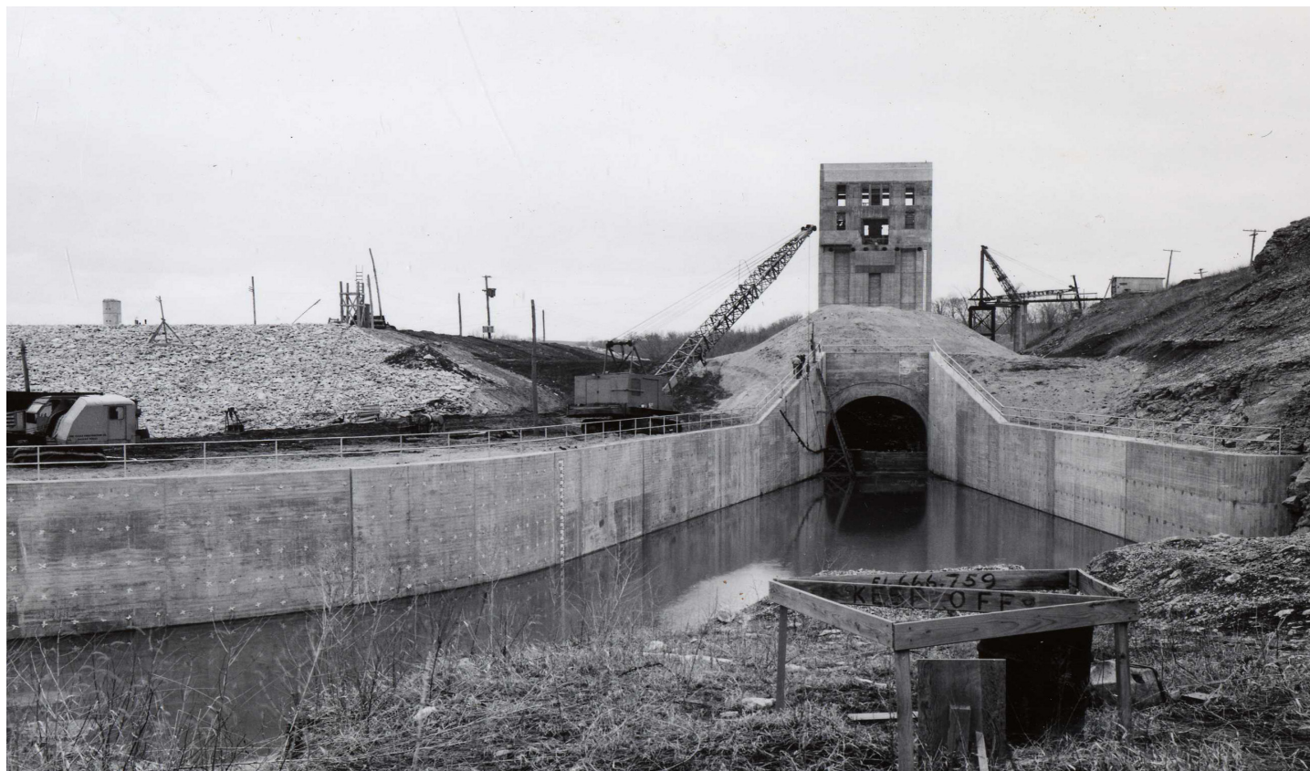
Looking north at construction of the outlet works and control tower for the Coralville Reservoir on the Iowa River in 1952. District Library Photo
