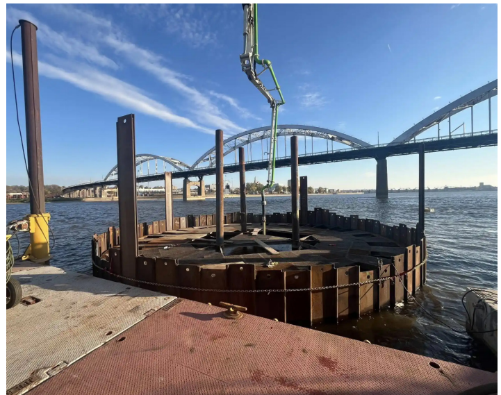
A mooring cell being constructed in Pool 16 of the Mississippi River as part of the Navigation and Ecosystem Sustainability Program. Photo by Vontrice Jones
