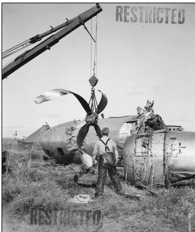
Figure 5: While training men to perform maintenance on the Boeing B-29 at Tinker, a mobile repair function was developed and utilized on downed aircraft.
