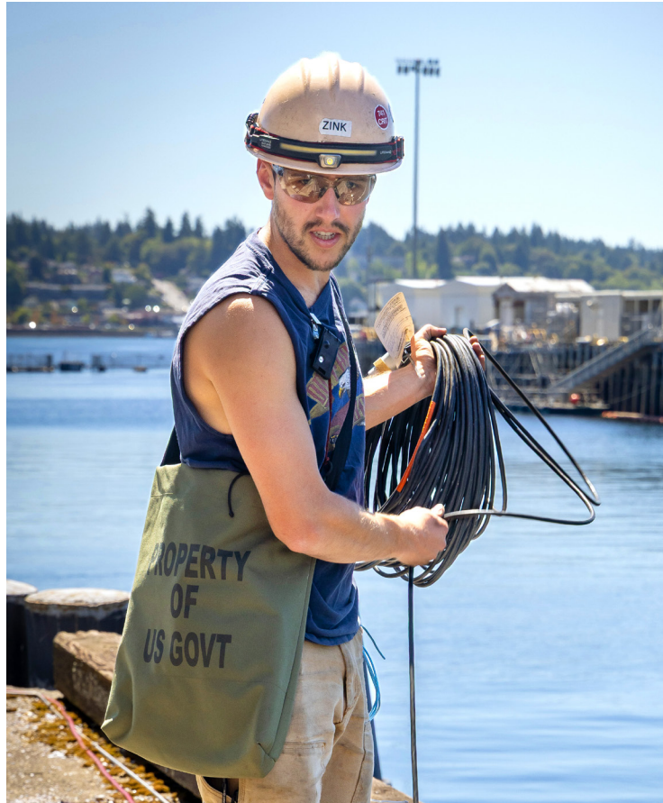
Jason Zink, Electrician, Shop 99, Temporary Services
