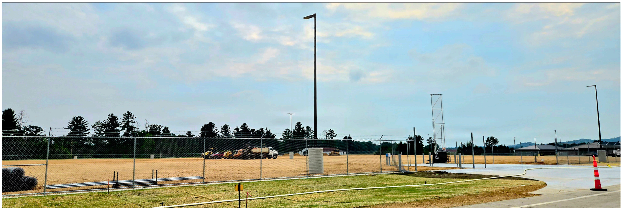
Workers with a contractor complete work Aug. 13 to construct a large parking area on the cantonment area for the at Wisconsin Maneuver Area Training Equipment Site at FortMcCoy.
