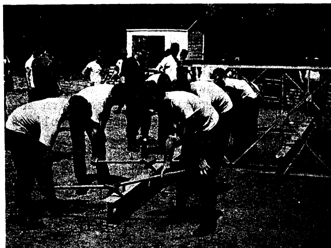
Members of the 972d Engineer Battalion assemble a Bailey Bridge during their annual training at Camp McCoy. (U. S. Army Photo)
