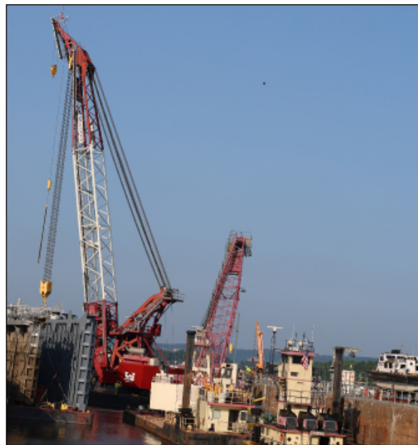
The miter gate replacement at Lock and Dam 9 near Lynxville, Wisconsin, July 21. USACE St. Paul District photo by Melanie Peterson
