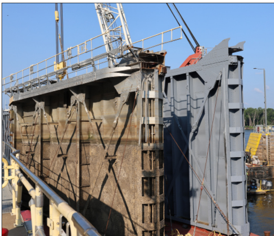
The old and new miter gates at Lock and Dam 9 in Lynxville, Wisconsin, July 21. USACE St. Paul District photo by Melanie Peterson
