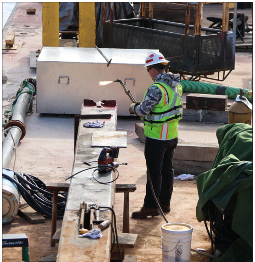
Jacob Jandl, marine machinery mechanic, cuts a piece of metal during the Lock and Dam 2 dewatering in Hastings, Minnesota, Feb. 14, 2024. USACE St. Paul District photo by Liz Stoeckmann
