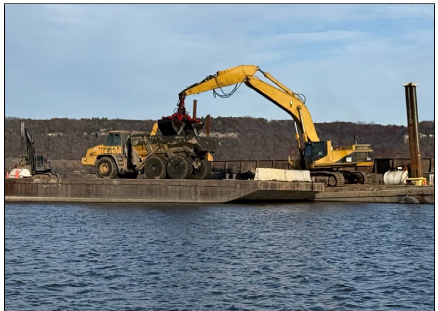
Construction continues on the Upper Pool 4 islands near Bay City, Wisconsin, Dec. 1, 2025. USACE St. Paul District courtesy photo
