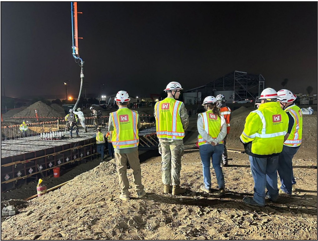
ABOVE: A newly placed concrete foundation cures June 30 at the site of a future aircraft hangar at March Air Reserve Base in Riverside County, California. The U.S. Army Corps of Engineers Los Angeles District is managing the construction of the facility to support the 452nd Air Mobility Wing's transition from the legacy KC-135 Stratotanker to the state-of-the-art KC-46A Pegasus.
