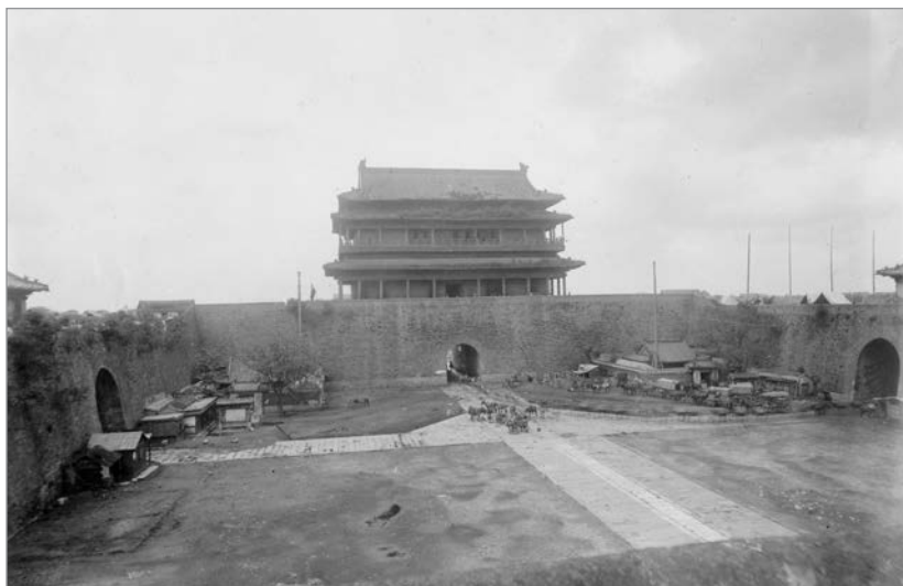
Rear of the Zhengyangmen. The walls are built double, creating a courtyard-like space between the inner and outer gate. (Upham, folder 11, Personal Papers Collection.)
