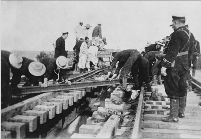
Sailors and Chinese workers repair a railroad. (NHHC, USN-901032.)
