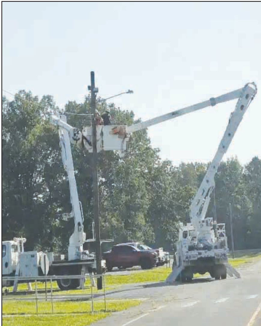
Photo above, Wes Hoffman and Ryan Garrett with Pine Bluff Arsenal's Directorate of Public Works-High Voltage Shop, work to restore the parking lot lights in front of the PBA Headquarters building. The lights were recently damaged due to a recent storm.
