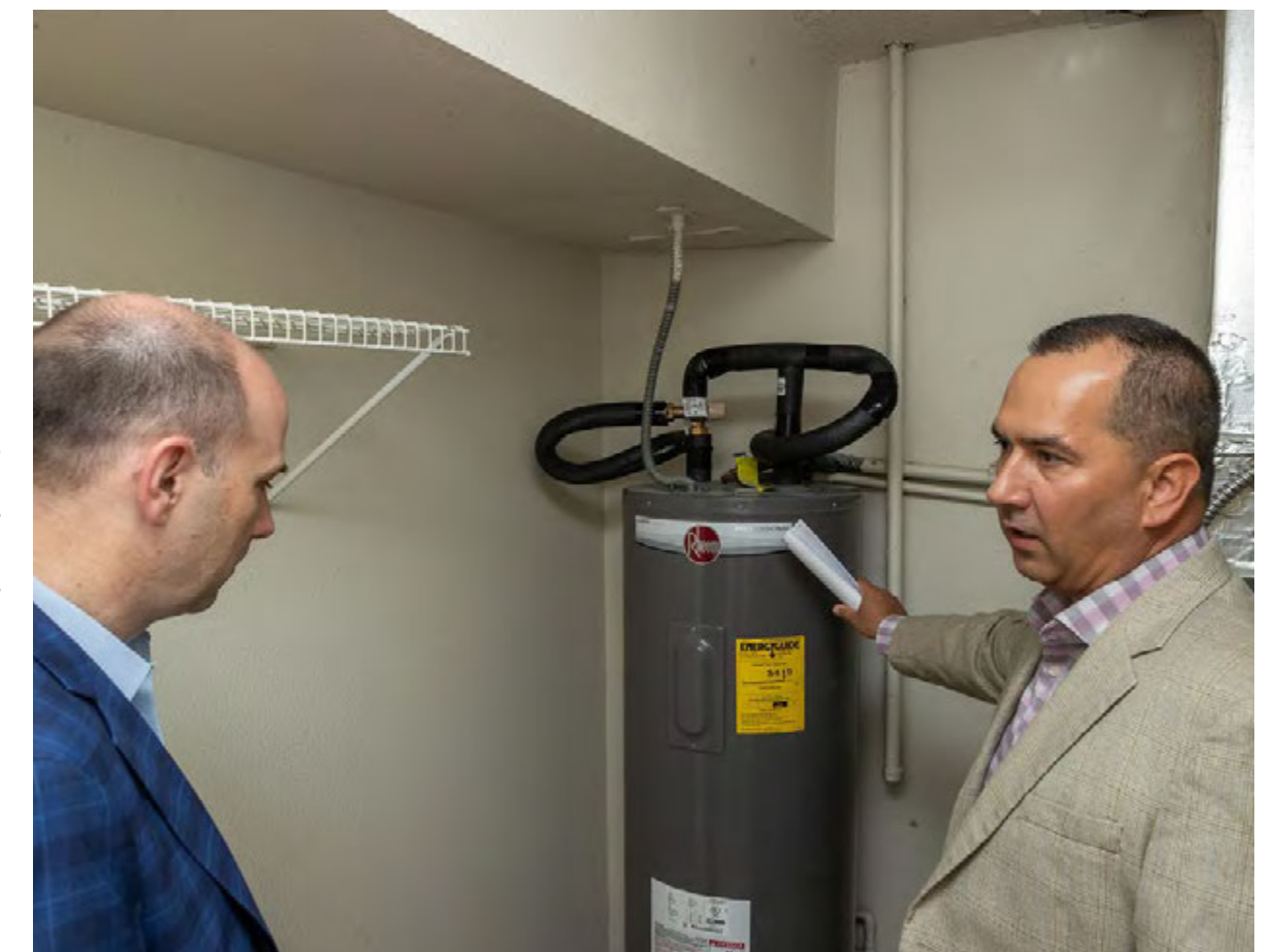
The Honorable Jordan Gillis, assistant secretary of the Army for installations, energy and environment, left, listens as Corvias Executive Vice President of Renewable Energy and Utilities Management Pablo Varela shows him one of Corvias' hot water system upgrades in a Palmetto Terrace home at Fort Polk, La., April 15. (U.S. Army photo by Porsha Auzenne)
