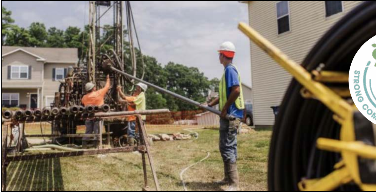
At Fort Polk, construction workers replace legacy HVAC systems with geothermal heating and cooling for more consistent indoor comfort and improved efficiency. (Courtesy Corvias)
