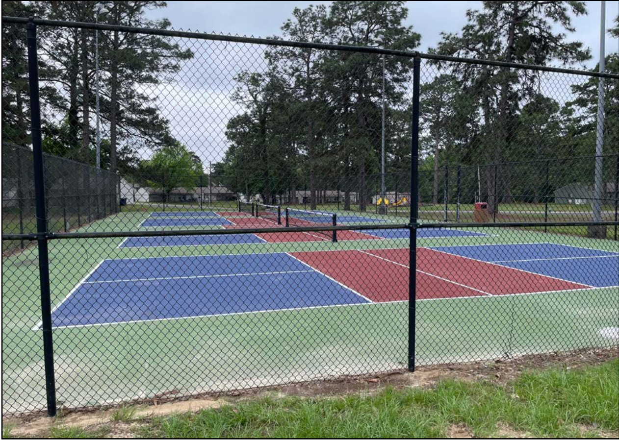
The Corvias pickleball courts are located on Seay St. in the Dogwood Terrace neighborhood. They are in the process of being completed. (U.S. Army photo by Angie Thorne.)
