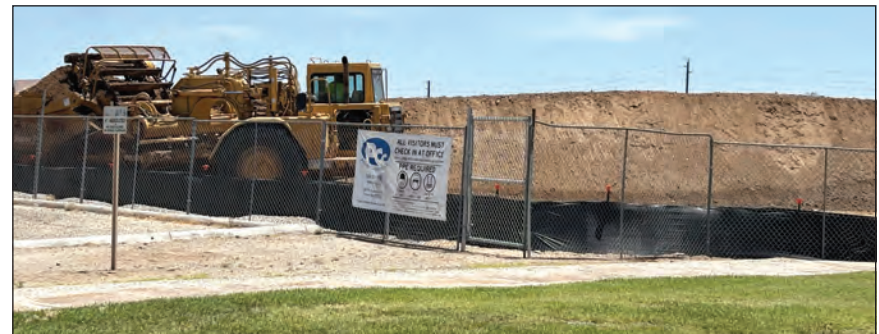
There is now visible progress on the construction of James D. Price Elementary School. Heavy equipment trucks are on site at the future home of the elementary school on post at U.S. Army Yuma Proving Ground (YPG). On May 19, YPG and Yuma Elementary School District #1 officials gathered for the ceremonial break ground on a new building for the school. The existing school building has served kindergarten through fifth grade youngsters on post since the 1950s (Photo by Ana Henderson)
