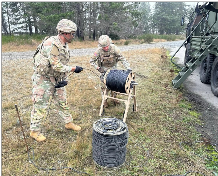
Staff Sgt. James Castilleja and Spc. Isaac Craig, 5th Battalion, 3rd Long Range Fires Battalion, 1st Multi-Domain Task Force, deploy tactical fiber-optic cable to establish secure communications between the Battery Operations Center and the Transporter Erector Launcher during training operations. (Photo by Sgt. Steven Andrade, 5-3 LRFB)
