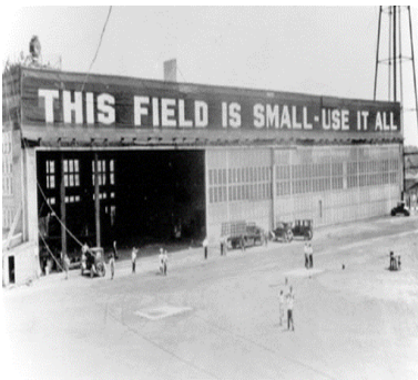
McCook Field main hangar.
