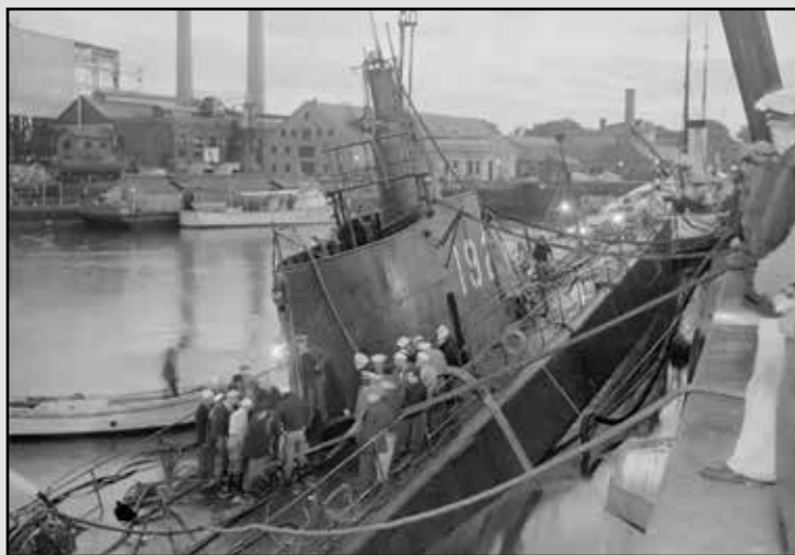
Squalus crew and shipyard workers pump water out of Squalus, at berth six, Portsmouth Navy Yard, September 14, 1939.
