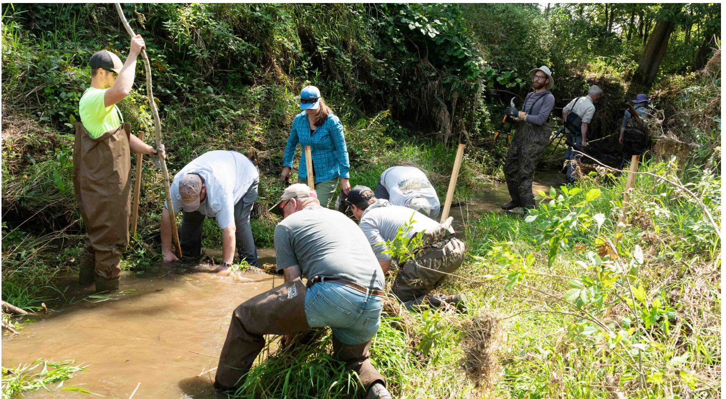
Volunteers pack in mud on top of the rocks to form the base of a beaver dam analog as the water levels begin to rise due to the introduction of branches and juvenile trees to form the outer walls. Photo by Jordan Raiff
