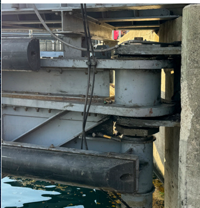
Left: Before repairing the pin, the assembly shown here was grinding metal-on-metal Photo by Mike Barry
