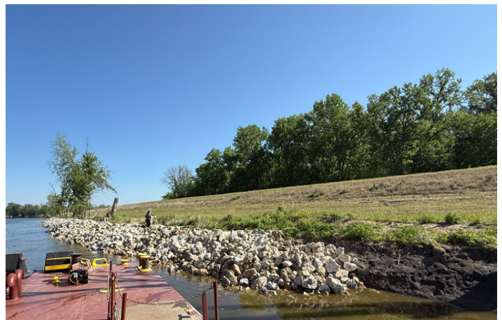
Before and after photos of levee repair work completed at the Bay Island Levee and Drainage District in Mercer County, Illinois. Photos courtesy of Emergency Management.
