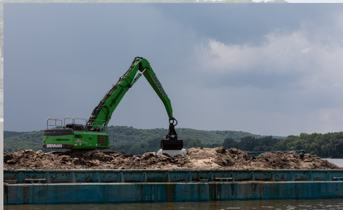
Chunks of debris and sediment are removed from the river bottom to make room for cofferbox construction.
