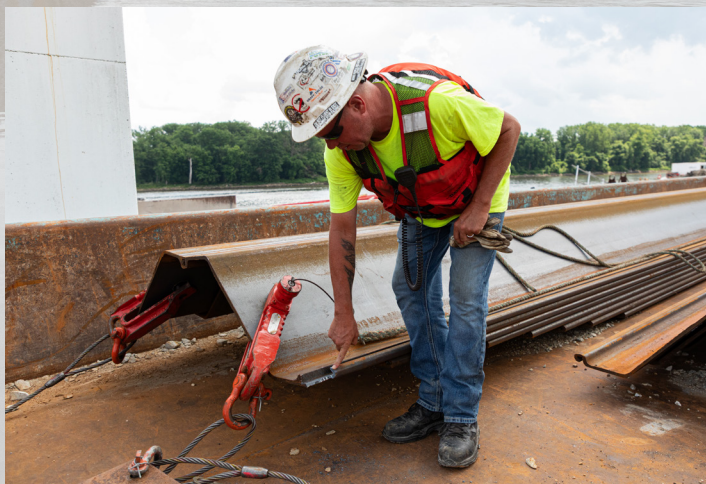
A member of the construction crew highlights a notch workers cut into the sheet steel for ease of installation without needing custom made steel. These sheets are being installed to create a cofferbox along the spillway. Once pumped out, workers will be able to work in the cofferbox to construct the fish ladder.
