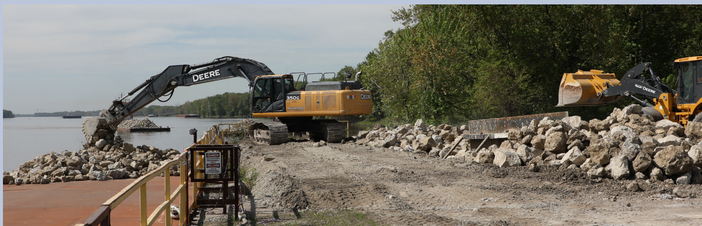
An excavator and loader move large rocks to a barge for transport to the Bay Island levee repair site near Lock and Dam 17 on the Mississippi River. Photo by Frances Candelaria
