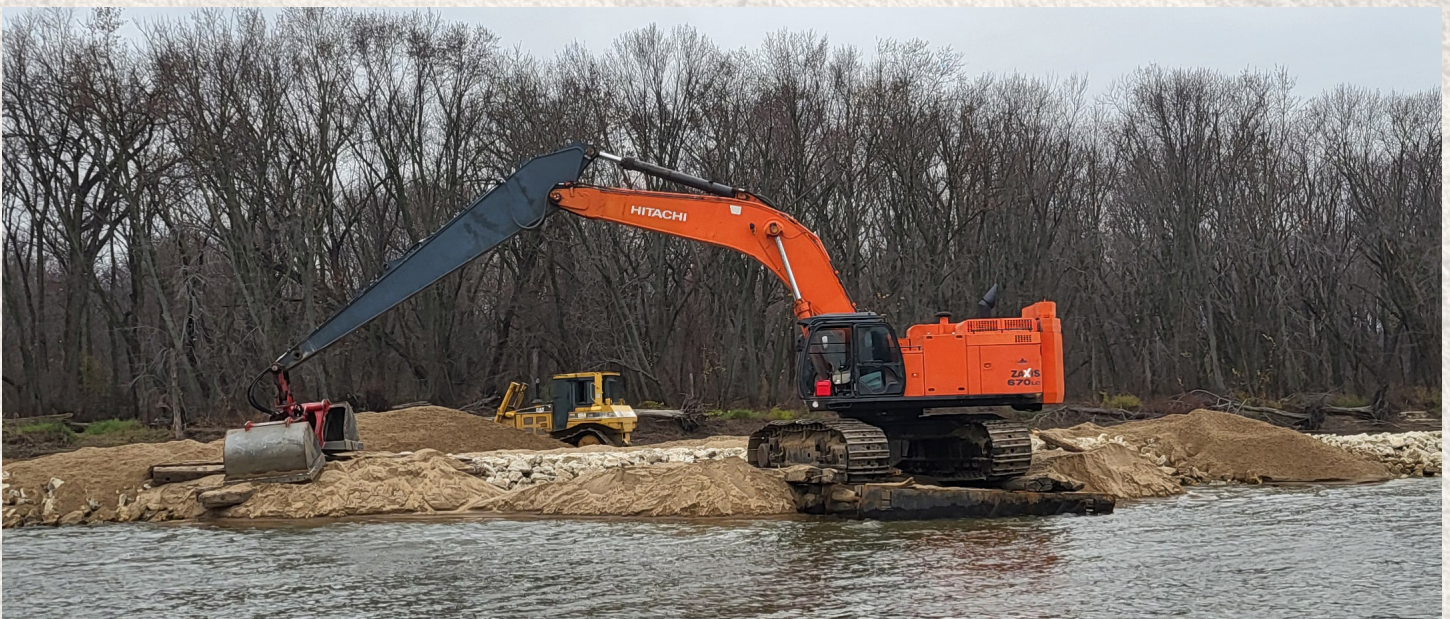
A contractor uses dredged material from the Rock Island District’s Beneficial Use Program to build up the head of Steamboat Island for an Upper Mississippi River Restoration – Habitat Rehabilitation and Enhancement Project near LeClaire, Iowa. Photo by Matthew Martin
