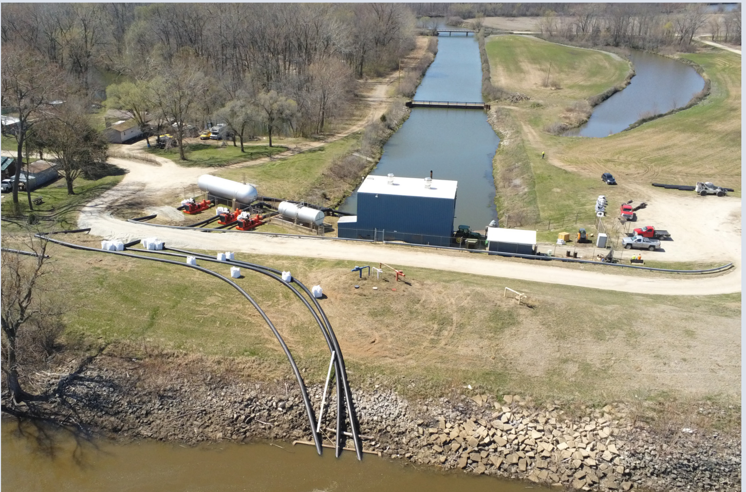
A view of the completed installation of emergency backup pumps and piping at the Muscatine Island Levee District-Louisa County Drainage District No. 13 Segment of the Muscatine, Iowa, Flood Risk Management System. Photo by Doug Vogel
