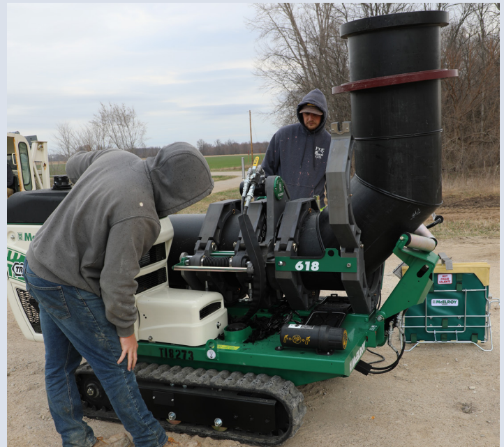
A specialized machine that uses a thermofusion process to connect high-density polyethylene pipes was used at the site to build a continuous leak-free system from the temporary 18-inch pumps to the river. Photo by Frances Candelaria
