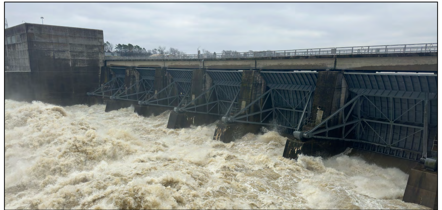
Old Hickory Dam in Hendersonville, Tennessee, releases 80,000 cubic feet of water per second Feb. 16 as part of flood control operations along the Cumberland River. USACE Nashville District estimates that USACE flood risk management projects prevented an estimated $734 million in flood damages across the Cumberland River Basin during February's heavy rainfall. (Photo by San Luciano Vera)
