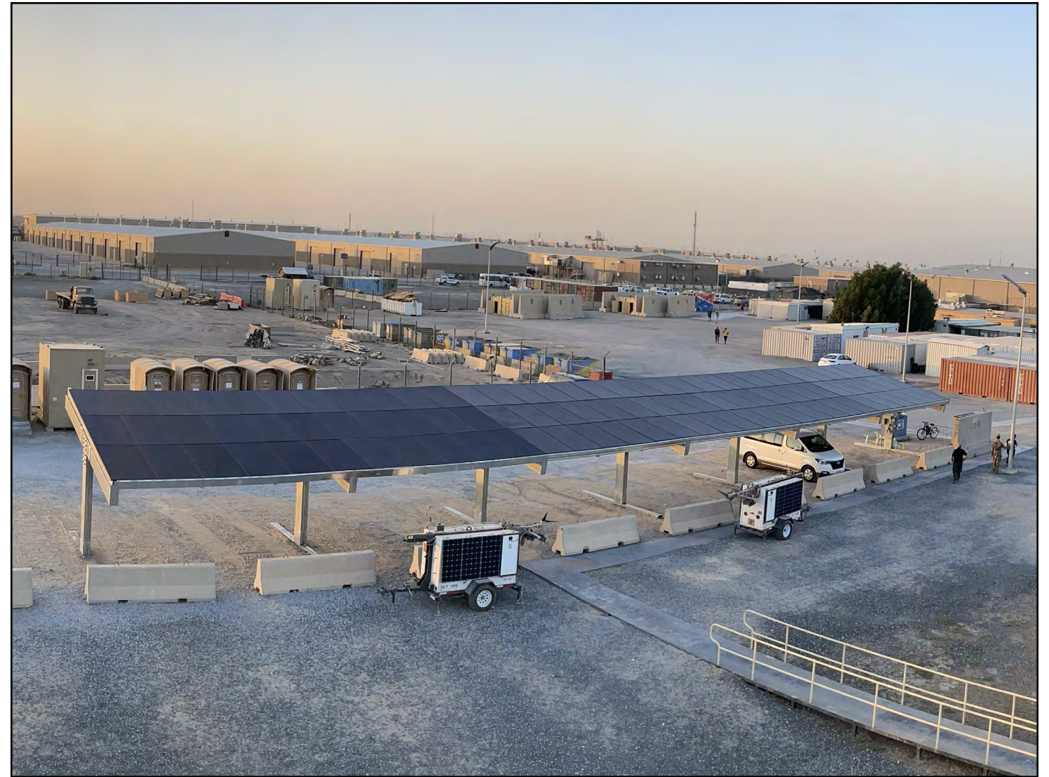
Camp Arifjan became a beacon of innovation and sustainability with the groundbreaking installation of a first-of-its-kind microgrid system in 2024. The microgrid provides balanced control of solar photovoltaic power and a large battery energy storage system. It also implements an improved utility grid connection architecture and integrates with a backup power plant and other control features, enhancing operational resilience and environmental sustainability while reducing noise pollution and fuel consumption. (Photo Courtesy of U.S. Army Central)
