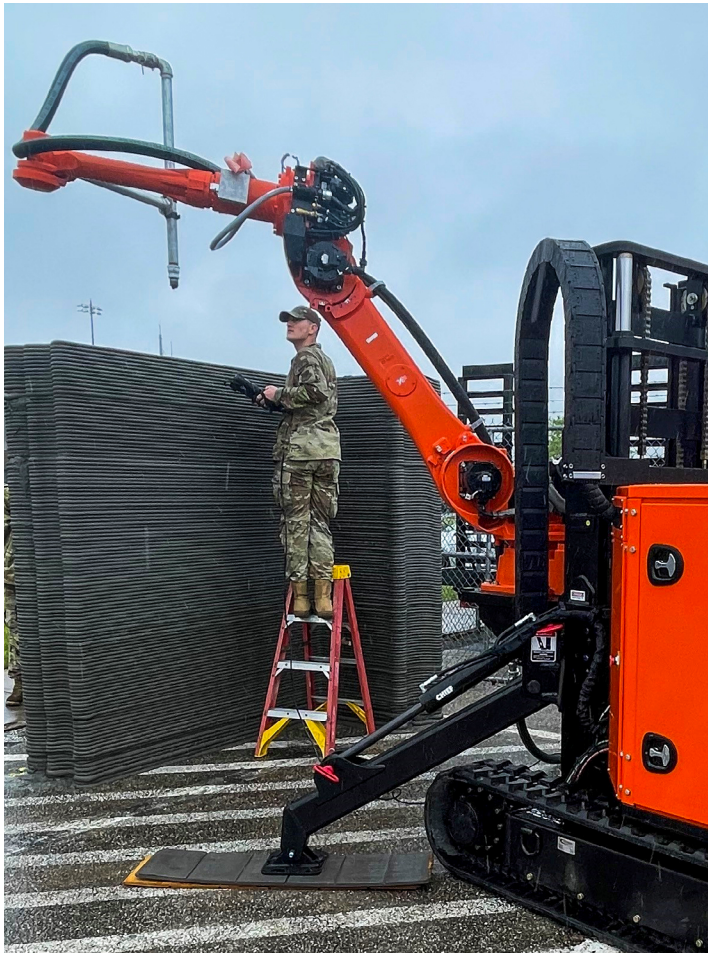
The 175th Civil Engineering Squadron at Warfield Air National Guard Base, Maryland, is at the forefront of innovation in developing an Expeditionary 3D Concrete Printer to rapidly build fortified infrastructure that supports warfighters and sustains operations in contested environments. (U.S. Air National Guard photo by Maj. Brian Vickers)
