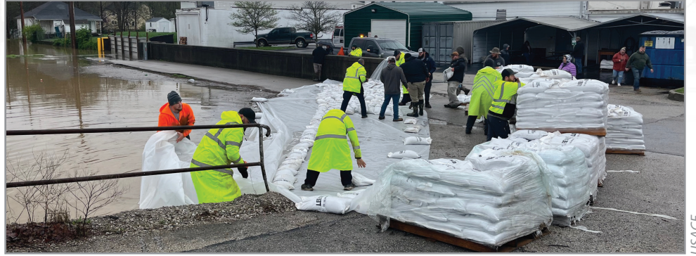
The Louisville District Flood Fight Teams from Levee Safety work with the local levee sponsors on sandbag placement in Frankfort, Kentucky, April 6.
