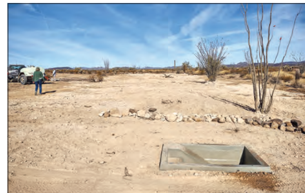
The wildlife drinker associated with the Red Raven Tank is meant specifically to help the Sonoran pronghorn continue its remarkable recovery efforts. "The shallow 26-inch trough will allow pronghorn to step in for a drink while still scanning the horizon for danger," said Daniel Steward, YPG Wildlife Biologist. (Loaned photos)
