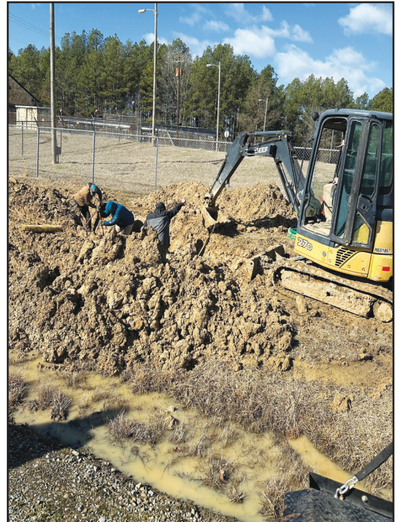
Scotty Bridges, Matt Newton, William Ives and Spencer Silvey with Pine Bluff Arsenal's Directorate of Public Works-Pipe Shop work to fix a broken gas pipe. U.S. ARMY PHOTO BY DPW
