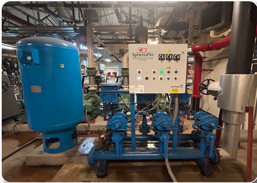
Replace Aft Sentry Village Booster Pump Bldg. No. 514
