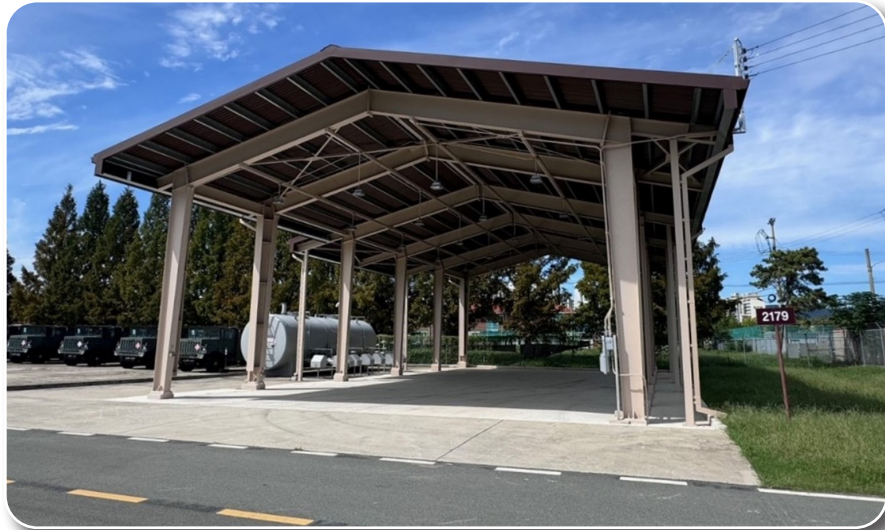
Construct Structural Steel Shade, Gwangju Air Base
