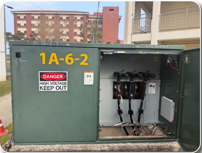
Replace T-Splice High Voltage Power Lines
