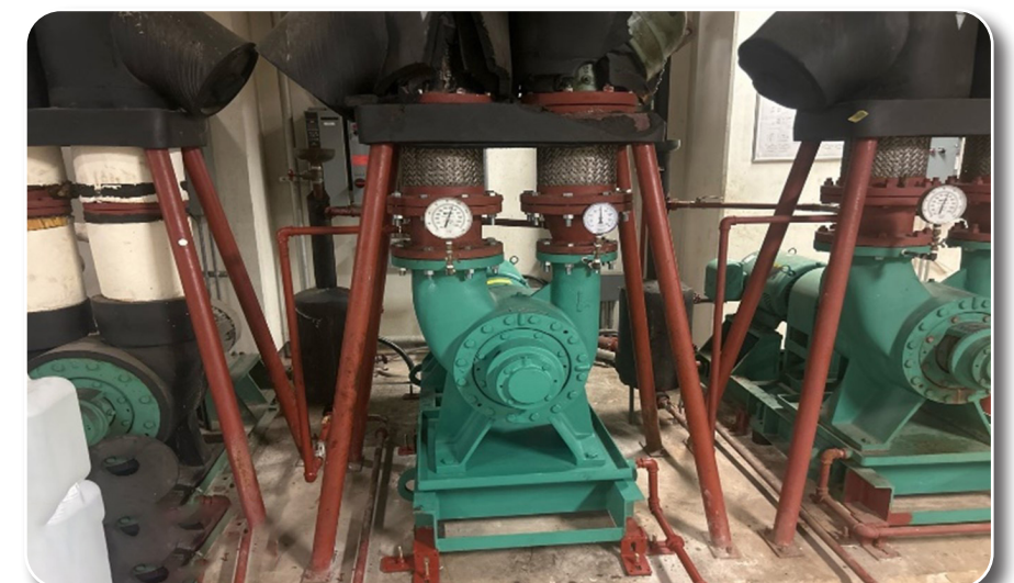
Replace 3 Double Suction Split Case Pumps Bldg. No. 5101, 5102 And 5103
