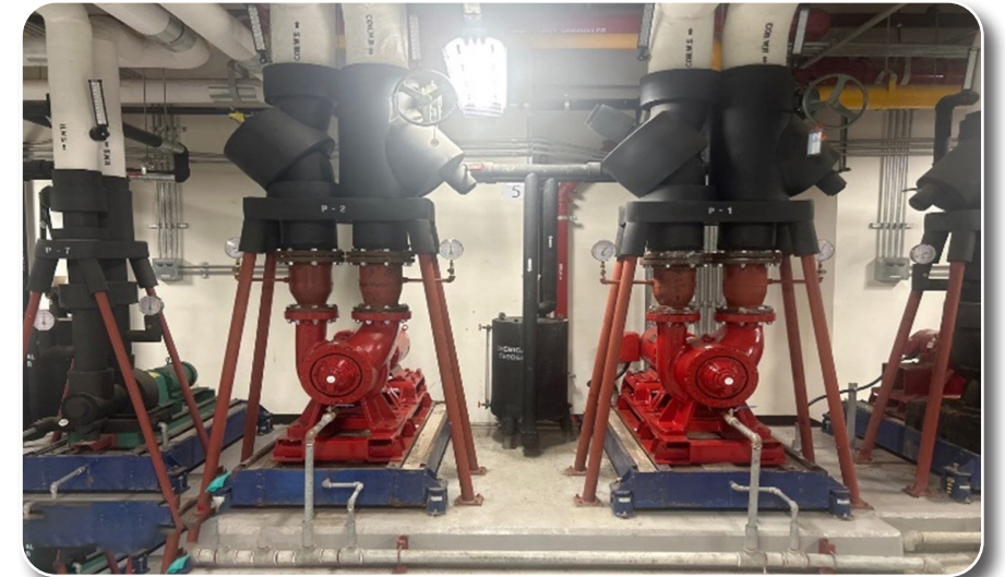
Replace 6 Double Suction Split Case Pumps and One Spare Bldg. 5171, 5172 and 5173
