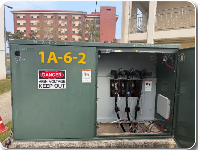
Replace T-Splice High Voltage Power Lines
