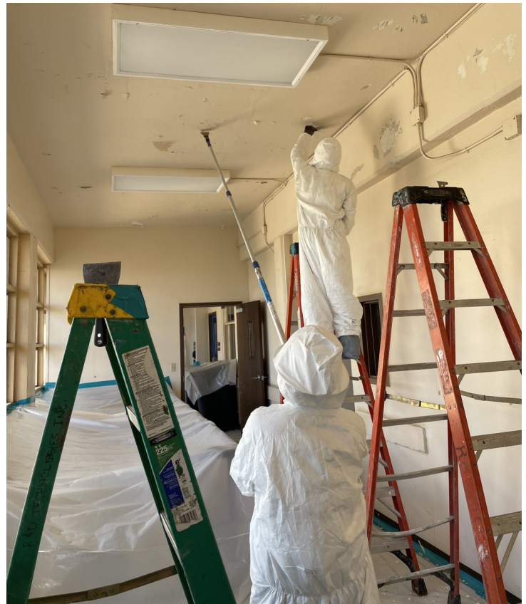
Crew members work to safely mitigate lead paint in preparation for painting. (Courtesy photo.)
