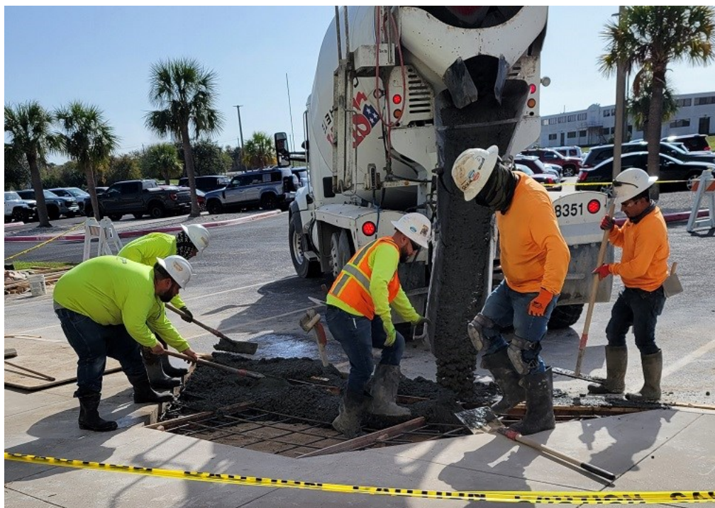
Construction crews pour concrete for accessible parking spaces at the Galveston District. (Courtesy Photo.)
