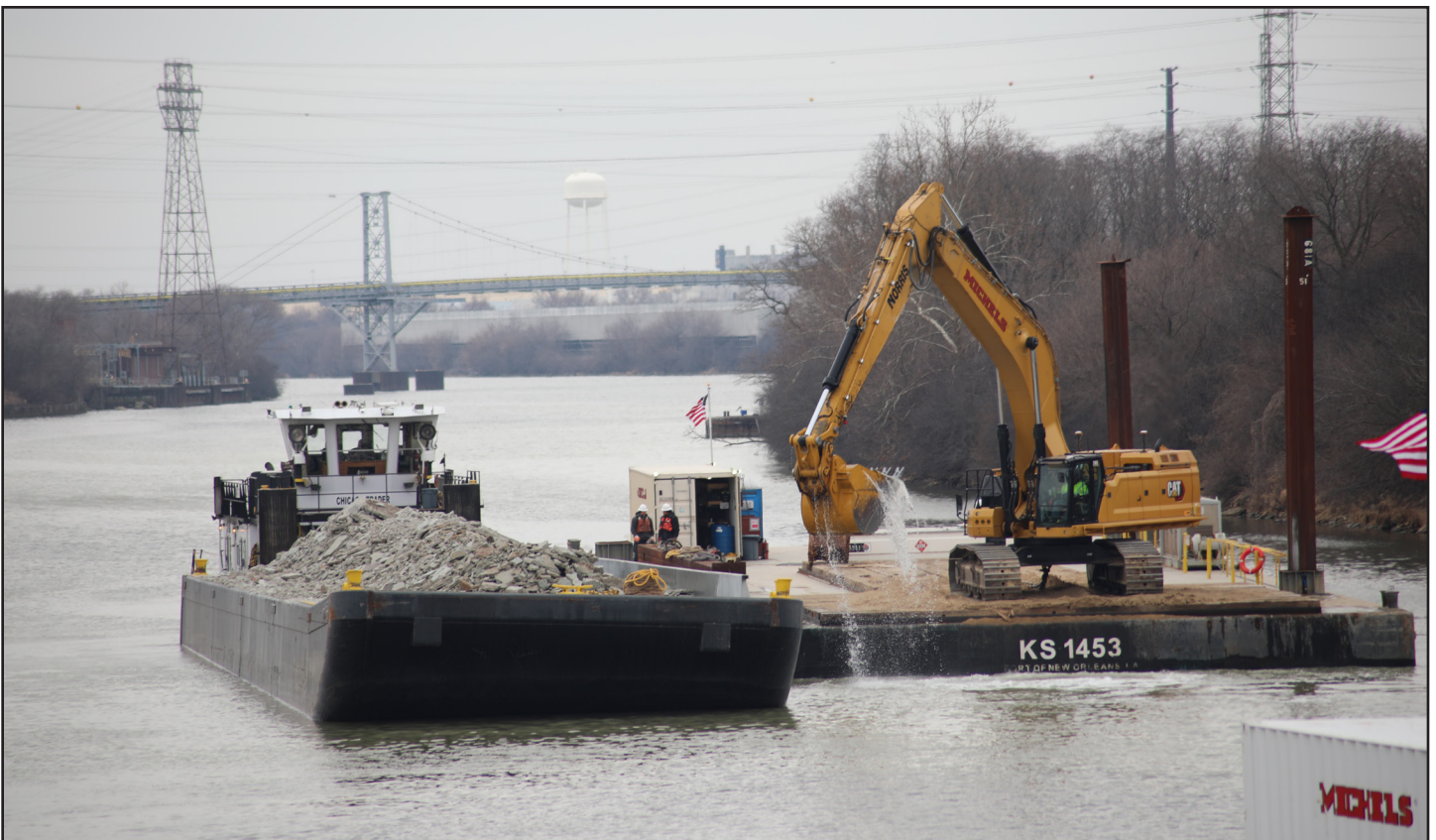
Contractors remove sand, silt and riverbed rock from the channel below the Brandon Rock Lock in preparation for construction of the Brandon Road Interbasin Project. Photo by Jim Finn
