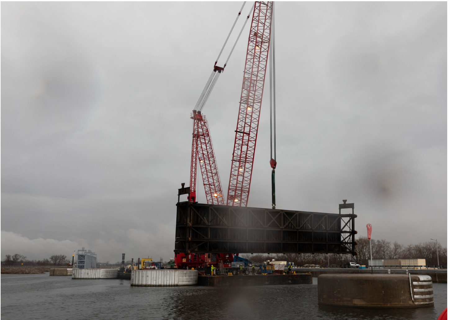
Crane operators remove the old gate from the Lockport lock. Photos by Jordan Raiff
