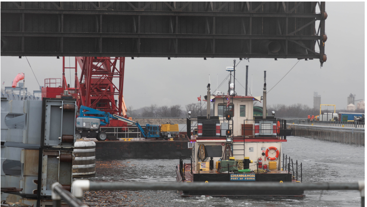
Crane operators remove the old gate from the Lockport lock. Photos by Jordan Raiff
