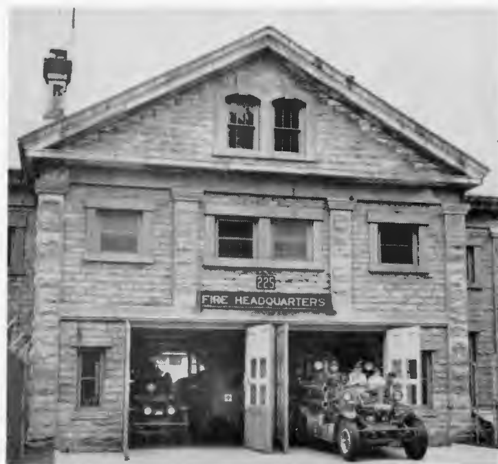
Ready for an alarm. Arsenal fire apparatus with hose rig manned.
