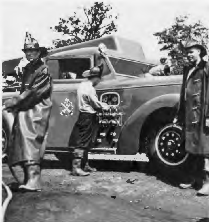
Modern fire fighting equipment. Compare with picture on page 28.
