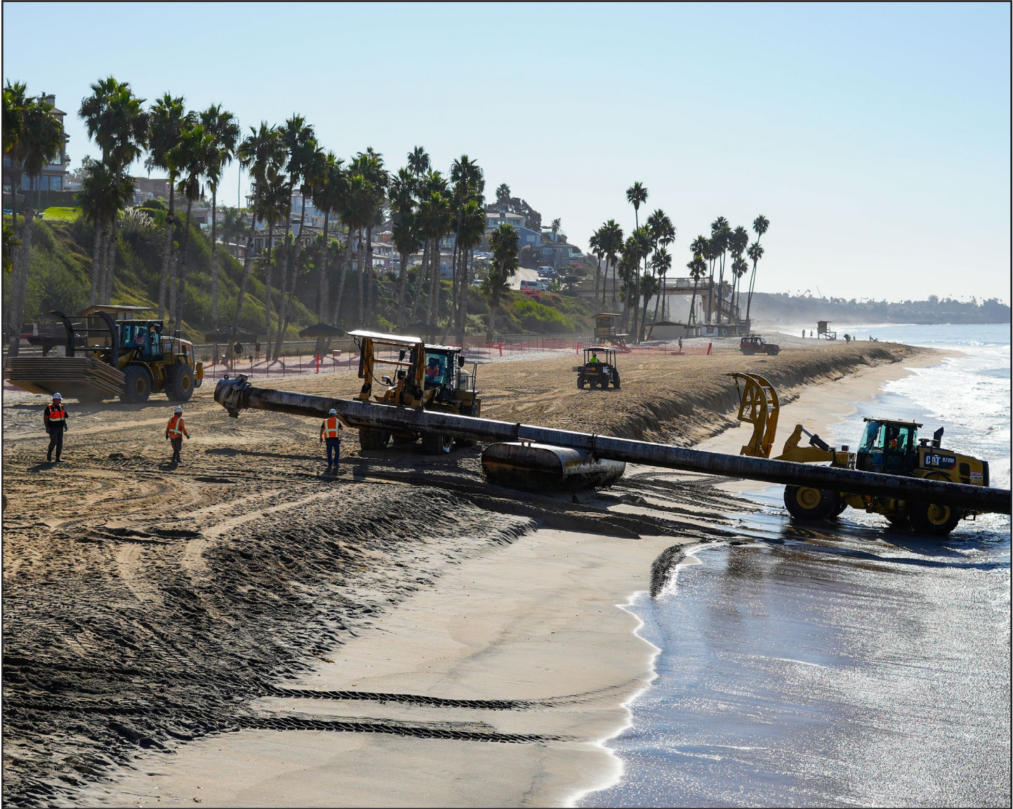
Contractors place a dredging pipeline onto the beach Oct. 31 in San Clemente, California.
