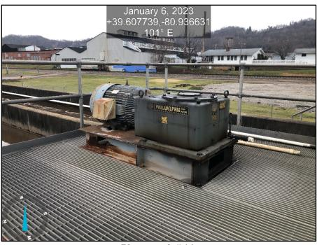
**Photograph # 14** WWTP, oxidation ditch pump
