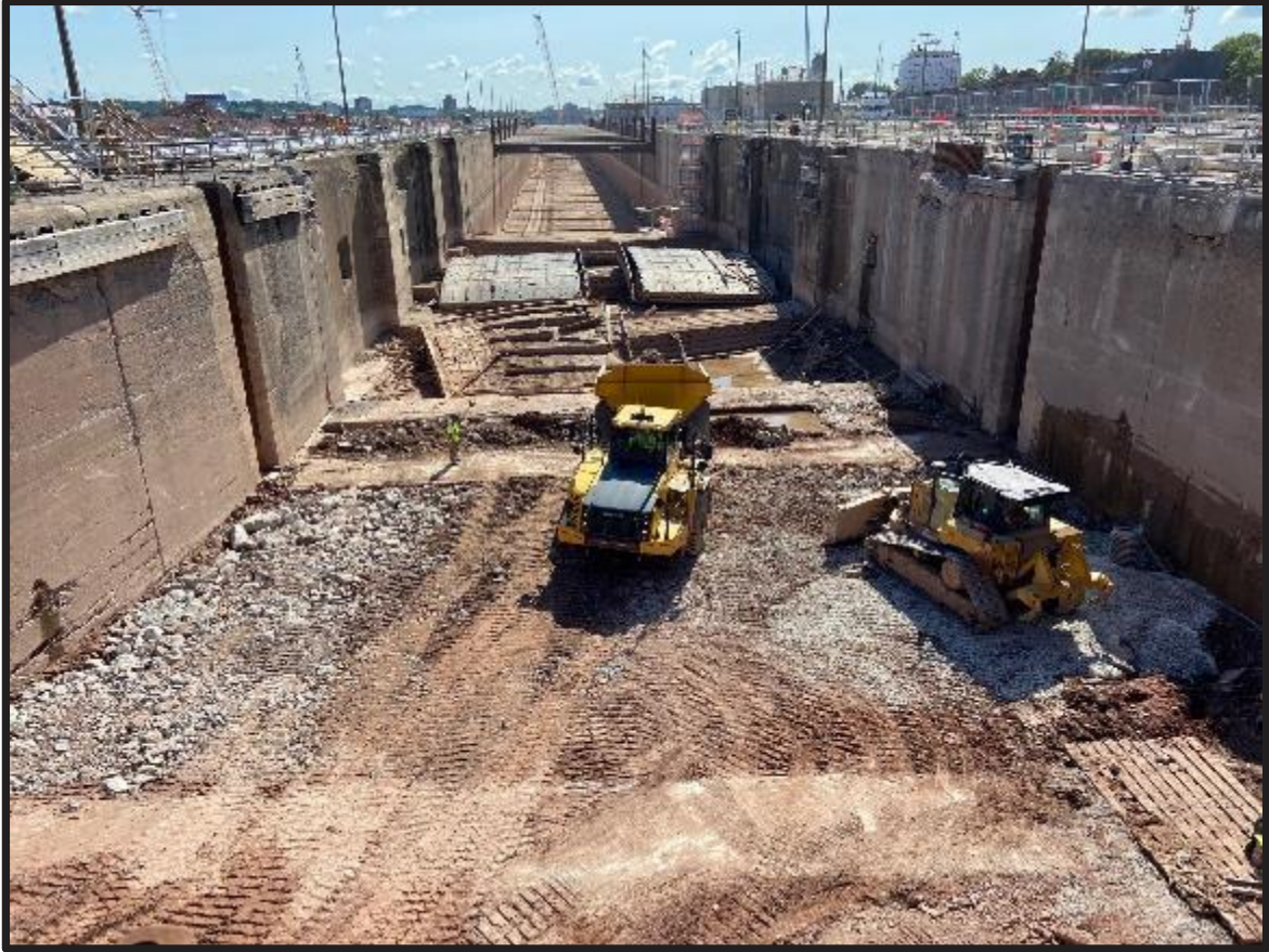
Placement of fill material in Davis Lock
