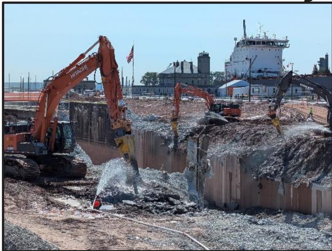
Middle of the Sabin Lock Chamber
