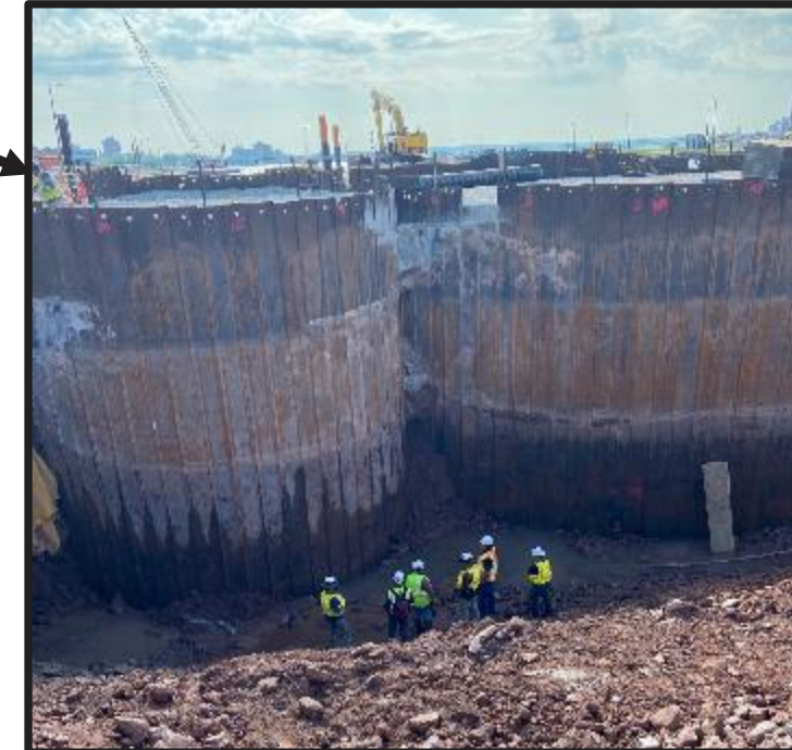
USACE inspection of the Downstream Cofferdam
