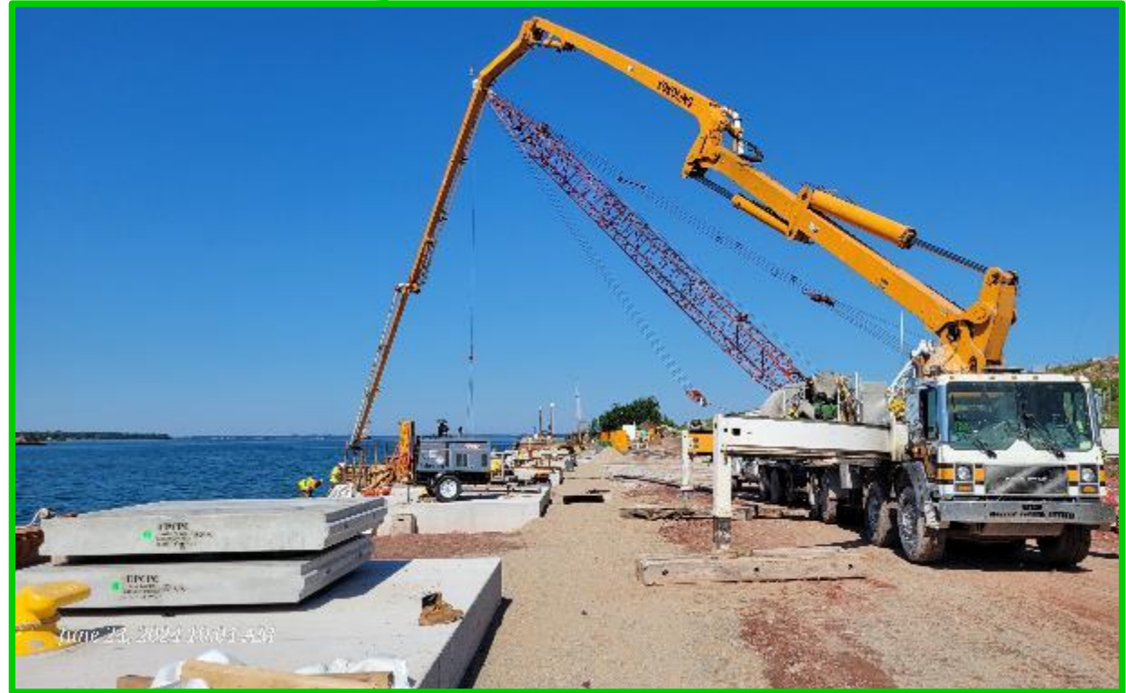
Placement of tremie concrete behind concrete panels
