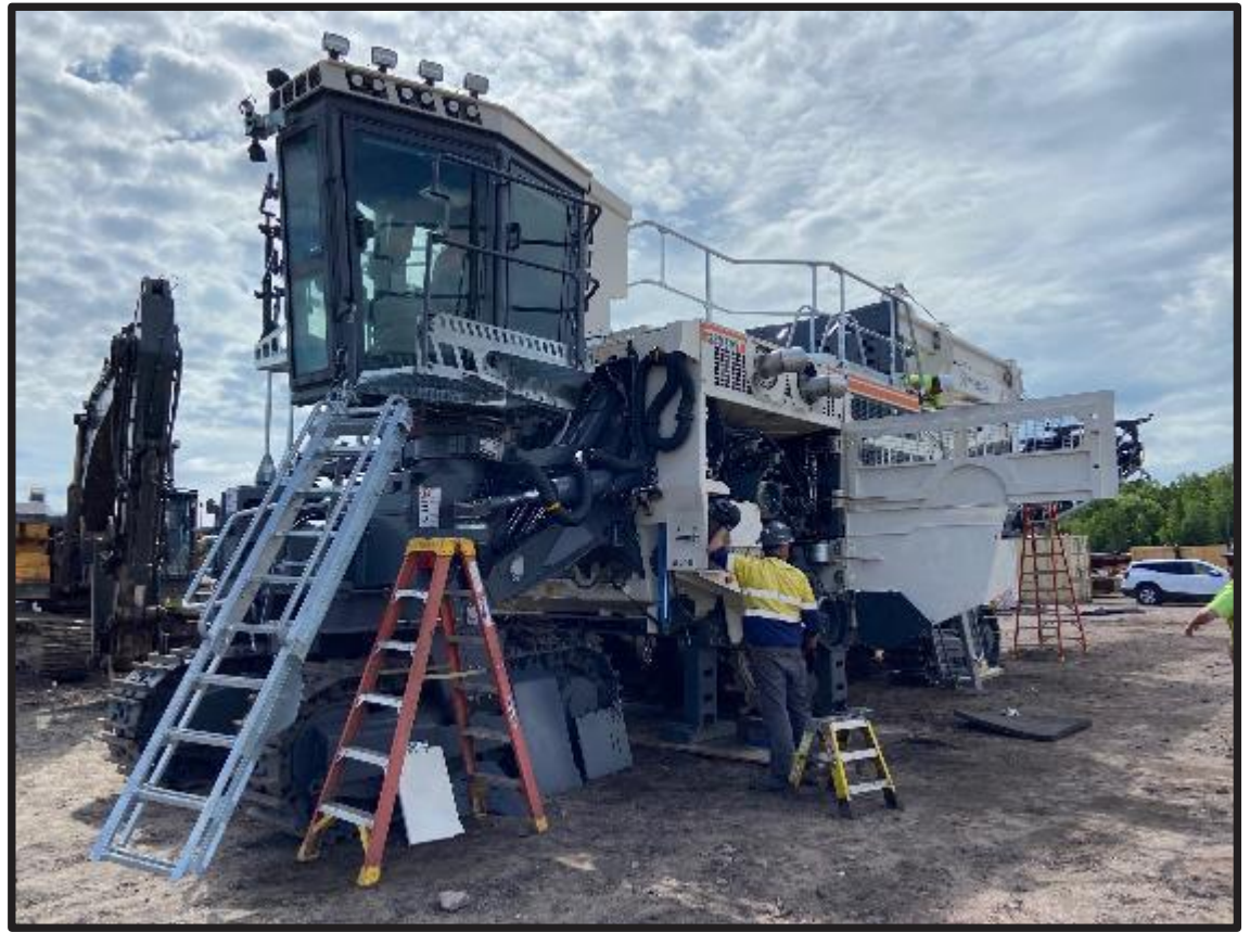
Assembly of Wirtgen milling machine to be used for bedrock excavation
