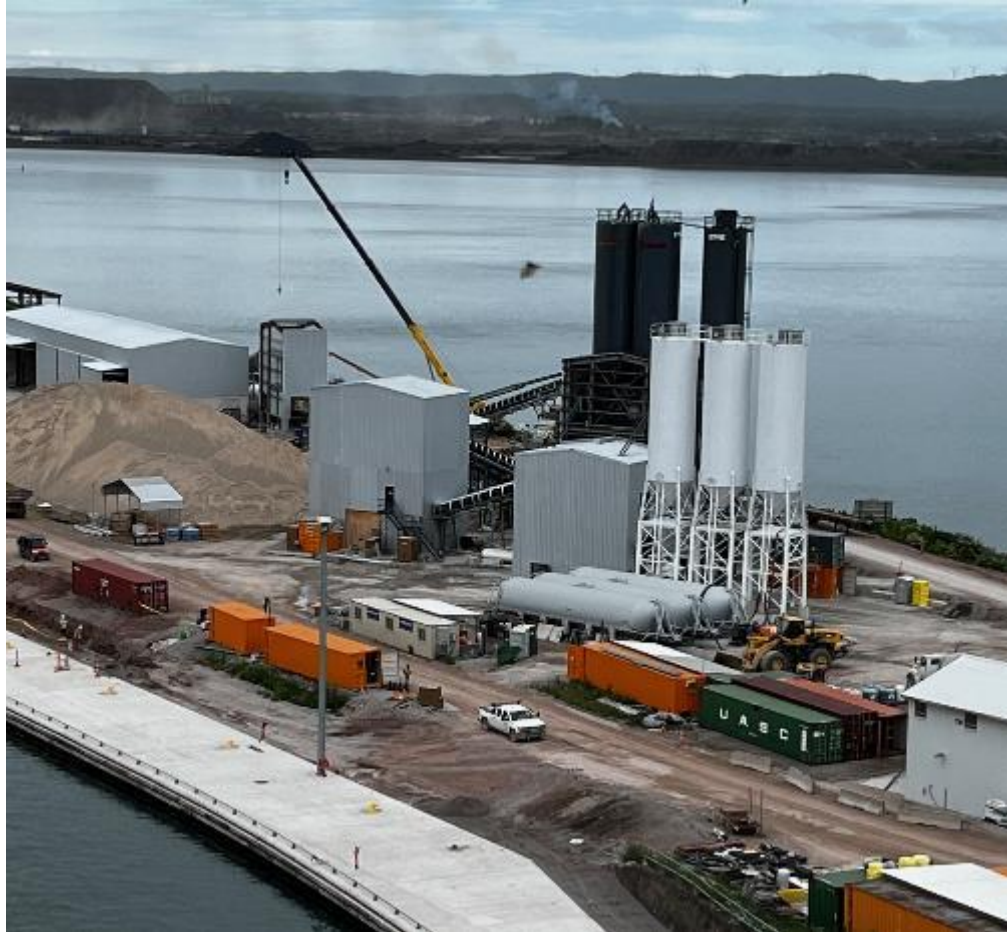
Concrete batch plant
