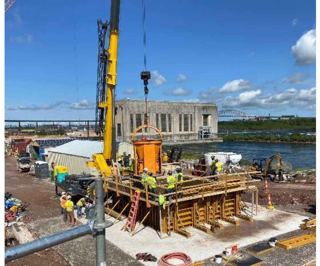
Placement of concrete in mass concrete test section
