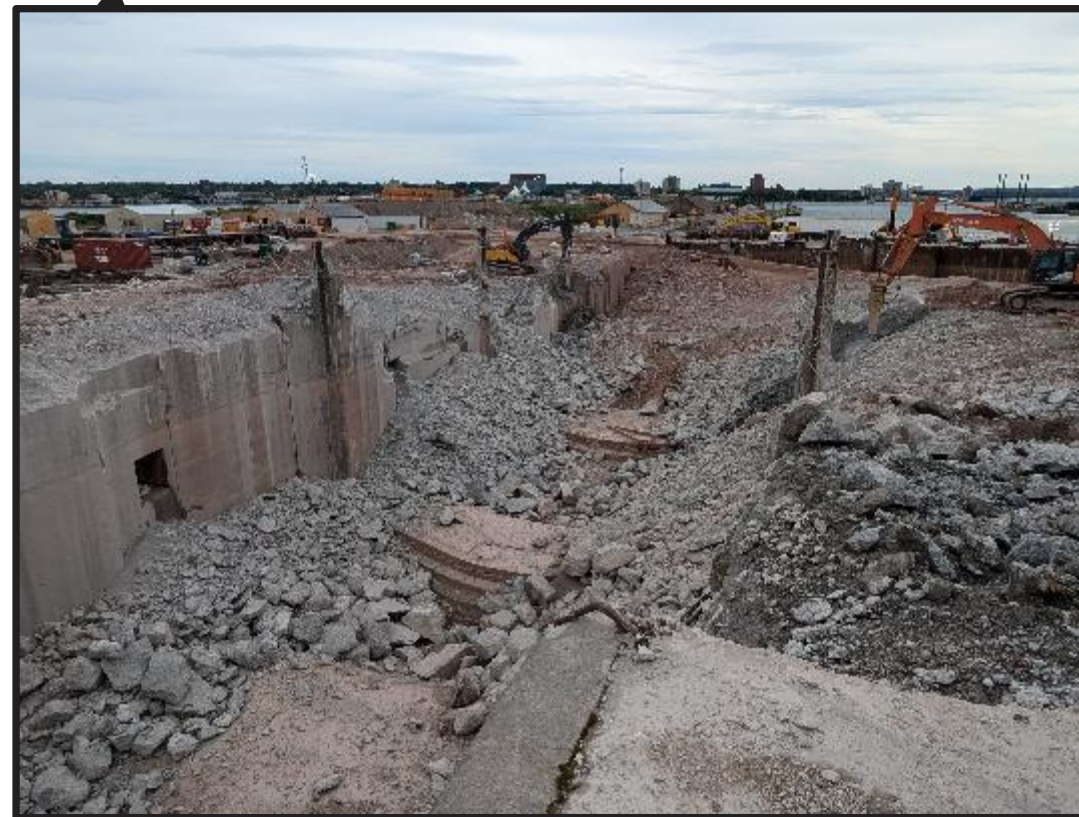
Downstream end the Sabin Lock Chamber
