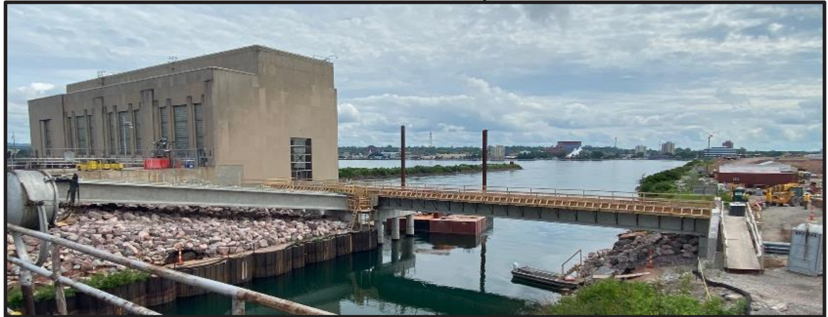
New bridge to the hydropower plant
