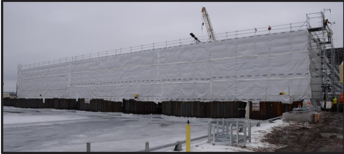
Upstream Cofferdam with Scaffolding Enclosure
