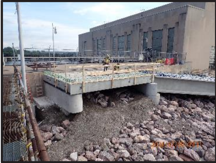
Connection of new bridge to landing at hydropower plant
