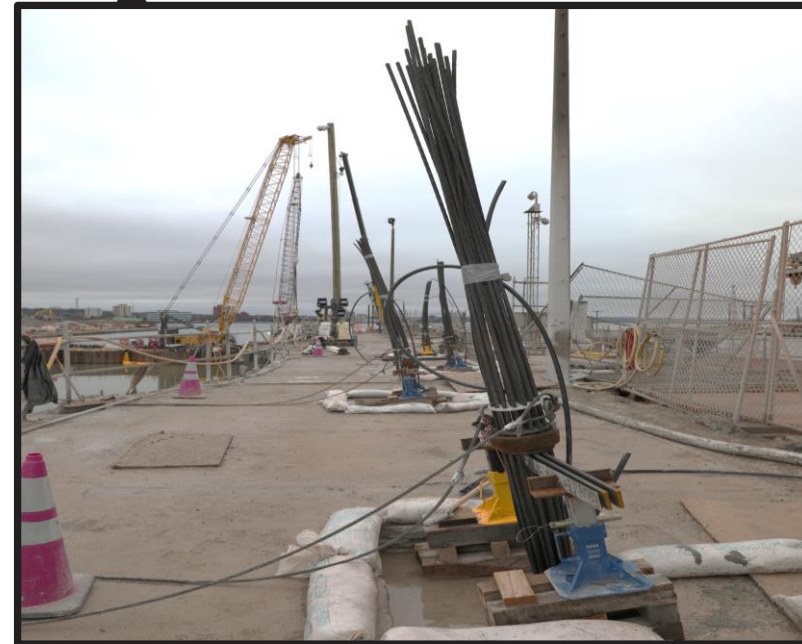
Rock anchor installation in Davis Lock monoliths
