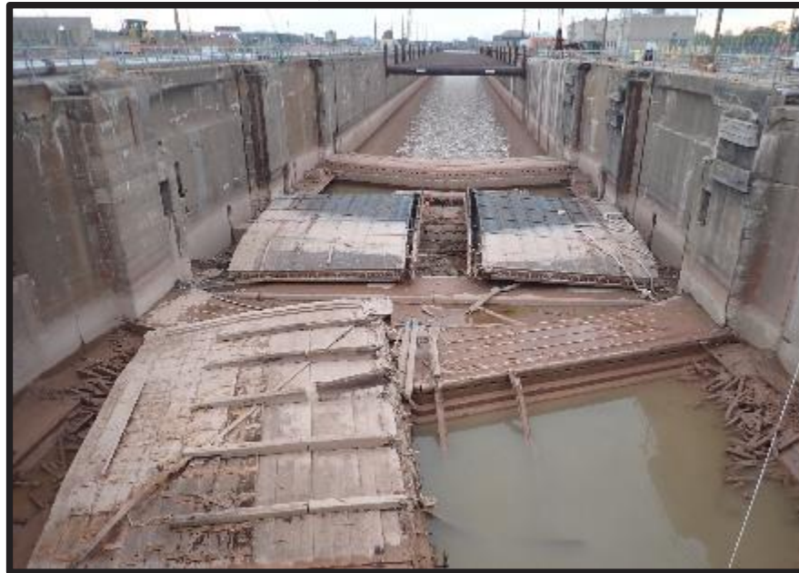
Davis Lock chamber five days into dewatering process
