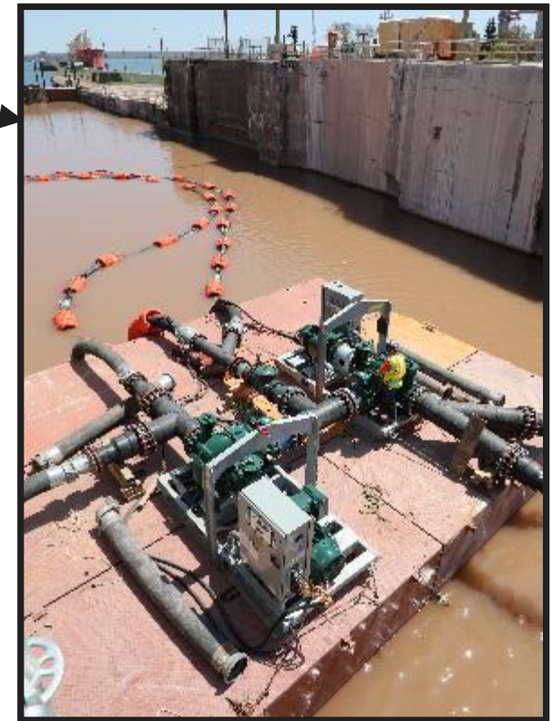
Hydraulic pump used to dewater construction site on barge in Davis Lock
