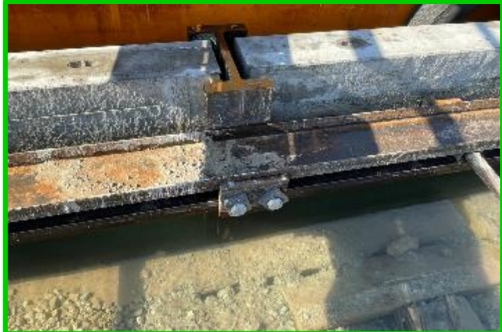
H-Pile, concrete panel, waler, and tie rod
