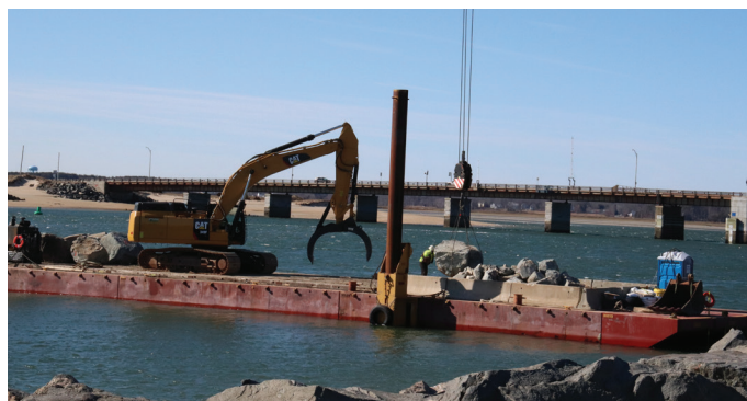
Contractor Lucianos Excavation moving armor stone for placement on the North Jetty.
