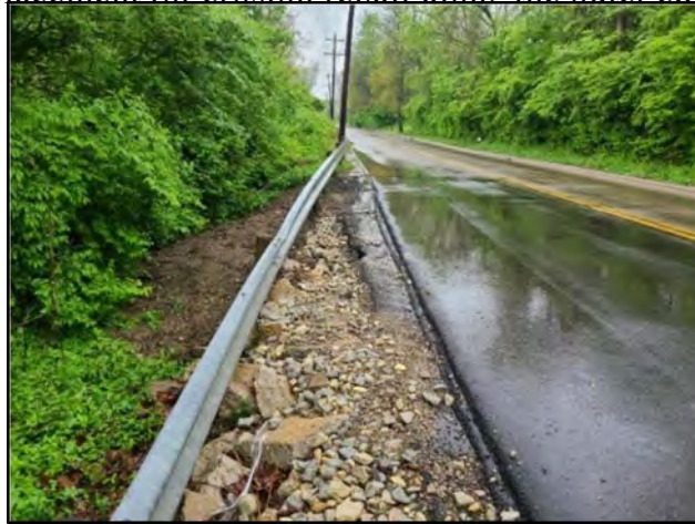
Figure 8: Displaced Guardrail and Asphalt Overlays at Site 1
