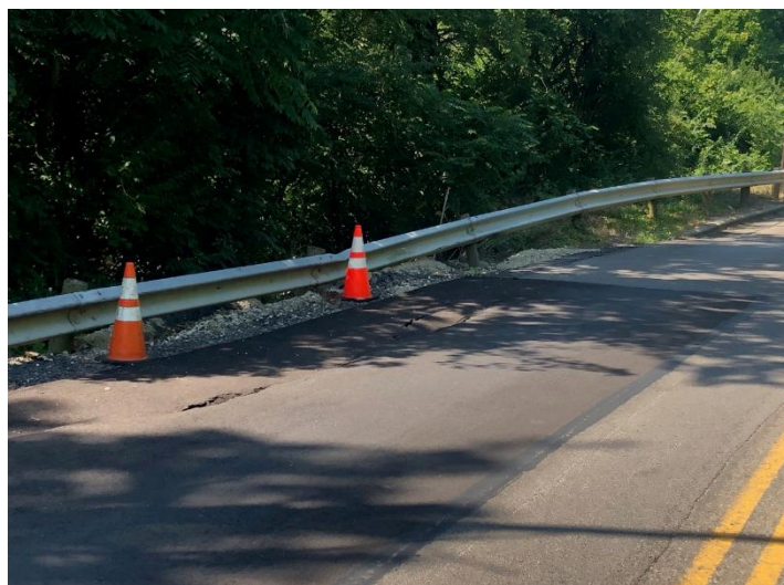
Figure 9 - Bank Failure Effect on E. Kemper Road in July 2023
