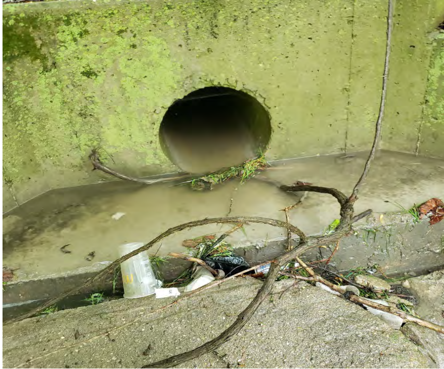
Photo 11 (Site 3): Silty sand soils observed in a storm sewer pipe at a headwall located on the slope between E. Kemper Road and Little Miami River (looking northwest).
