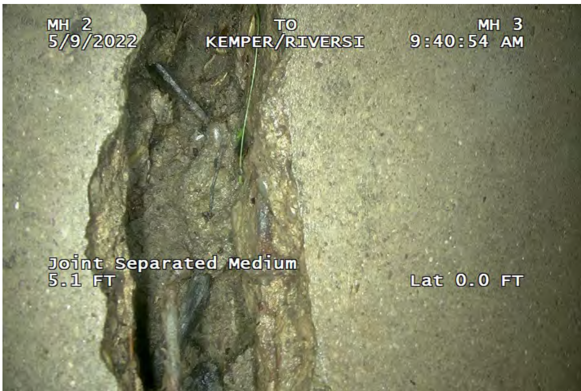
Photo 2 (Site 1): Joint separated at 5.1 feet between CB-2 and HW-3.
