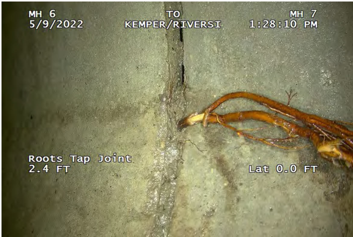
Photo 3 (Site 2): Roots tap joint at 2.4 feet between IN-6 and MH-7.
