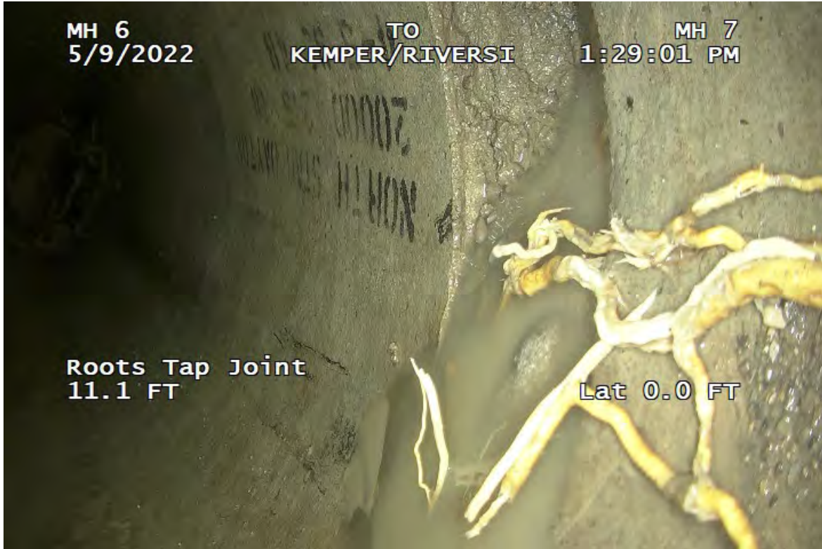
Photo 4 (Site 2): Roots tap joint at 11.1 feet between IN-6 and MH-7.
