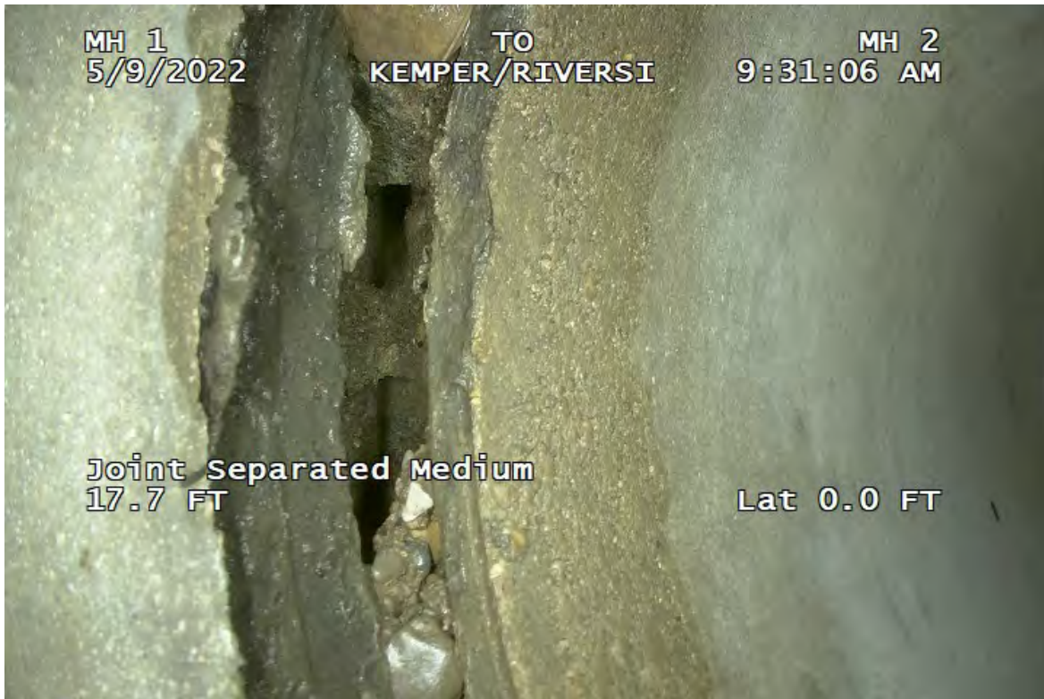
Photo 1 (Site 1): Joint separated at 17.7 feet between CB-1 and CB-2.
