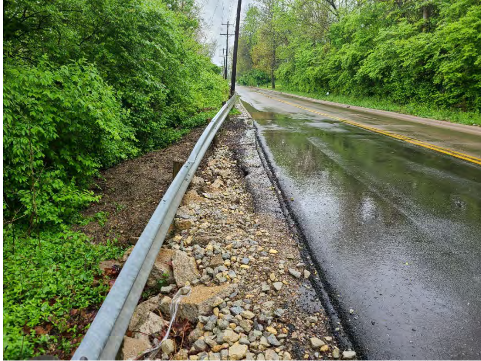
Photo 1 (Site 1): Guard rail movement, asphalt settlement and resurfacing, and stone placement for erosion repair on the southeast side of E. Kemper Road (looking southwest).
