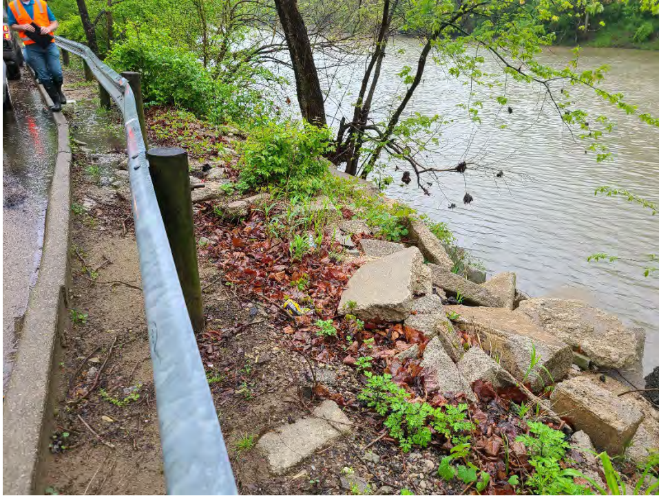
Photo 5 (Site 2): Stone/concrete debris placement on slope between E. Kemper Road and Little Miami River (looking northeast).
