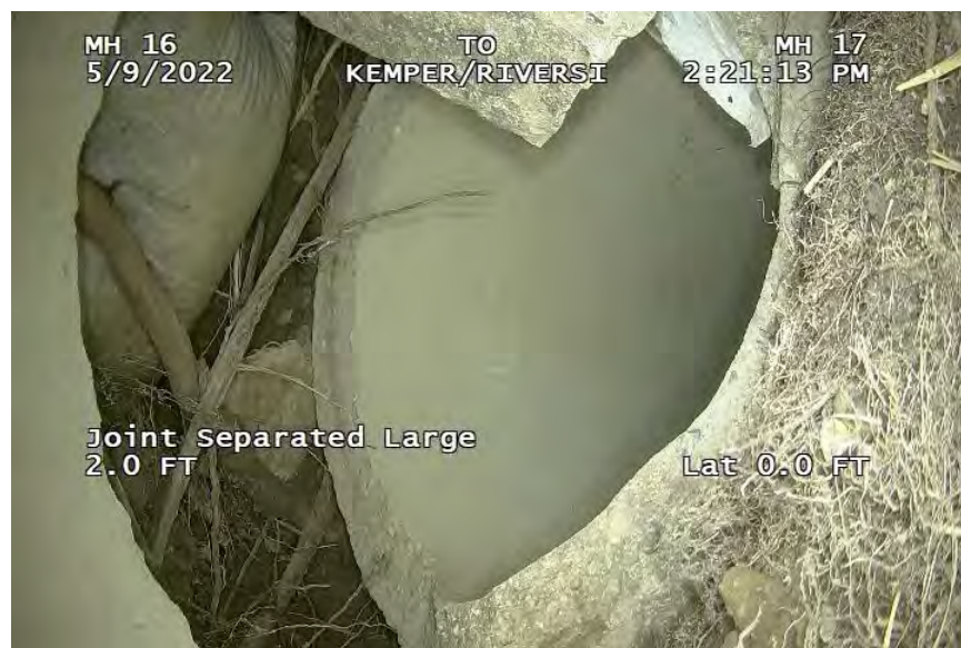
Figure 13: Joint Separation at Site 3
