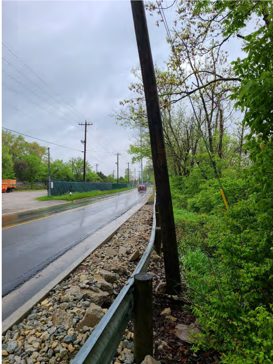
Photo 8 (Site 3): Guard rail movement, leaning light pole, and stone placement for repair on the southeast side of E. Kemper Road (looking northeast).
