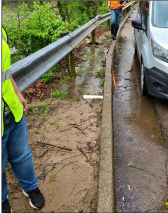
Figure 9: Small Drainage Pipes Penetrating the Curb on the Southeast Side of E. Kemper Road
