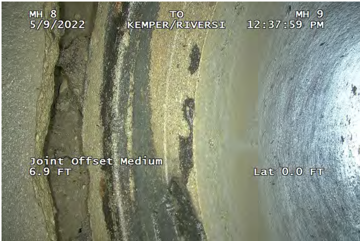
Photo 7 (Site 2): Joint offset at 6.9 feet between CB-8 and HW-9.
