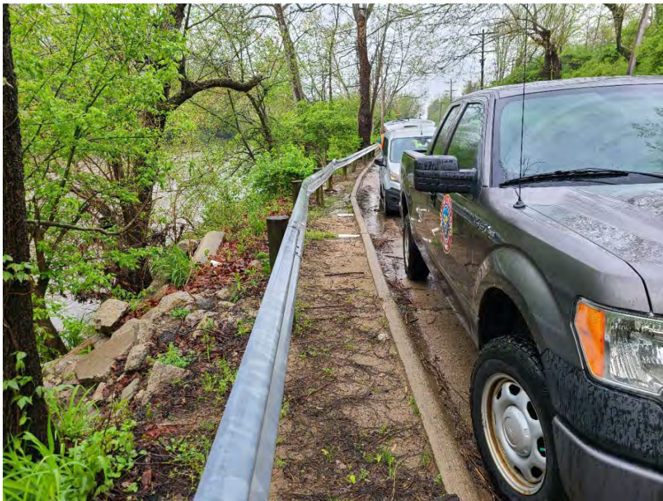
Photo 6 (Site 2): Small drainage pipes penetrating the curb on the southeast side of E. Kemper Road and leaning tree (looking southwest).
