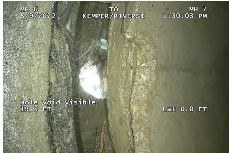
Figure 12: Joint Separation with hole Visible to Surface at Site 2
