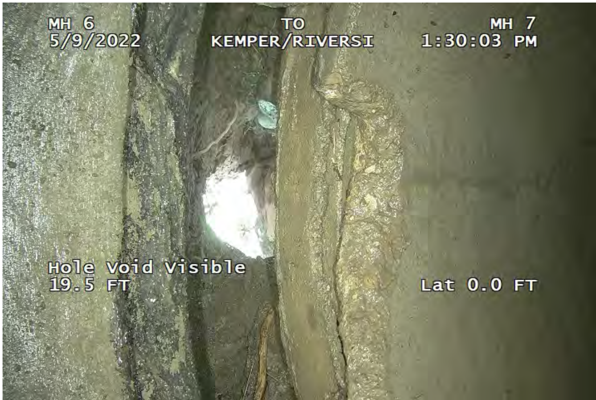
Photo 5 (Site 2): Hole void visible at 19.5 feet between IN-6 and MH-7.
