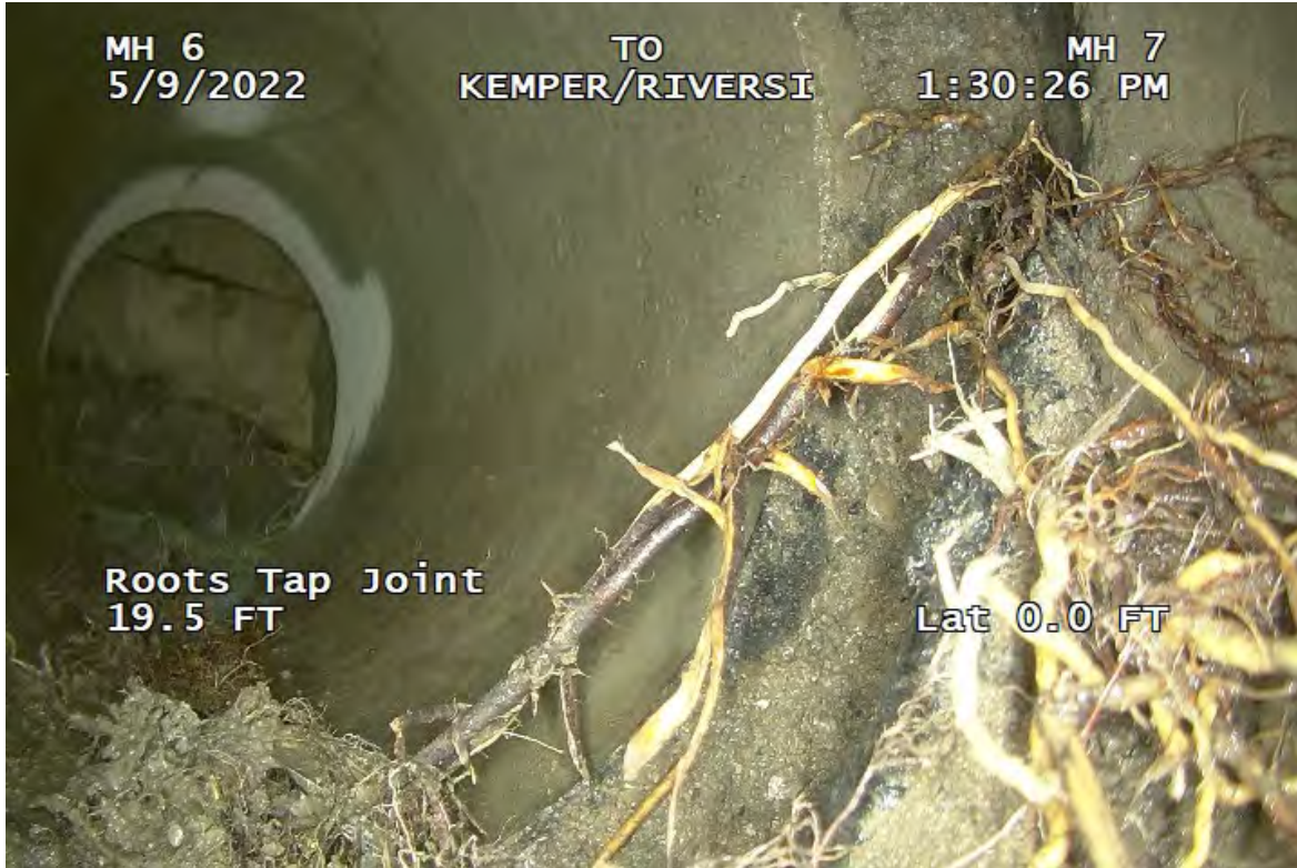
Photo 6 (Site 2): Roots tap joint at 19.5 feet between IN-6 and MH-7.
