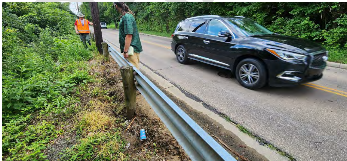
Figure 7: Little Miami River, Loveland, OH Work Site 1 (Downstream site) illustrating tension cracks at the edge of the roadway/guardrail.
