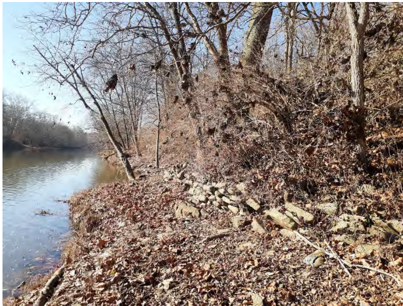
Figure 10: Dry laid limestone terrace at northeast edge of Site 2 (looking southwest)
