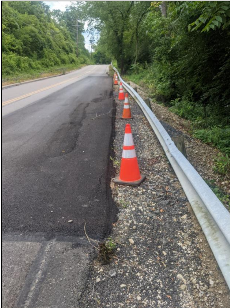
Photo above shows an area experiencing slope failure along E. Kemper Road in Loveland, Ohio
