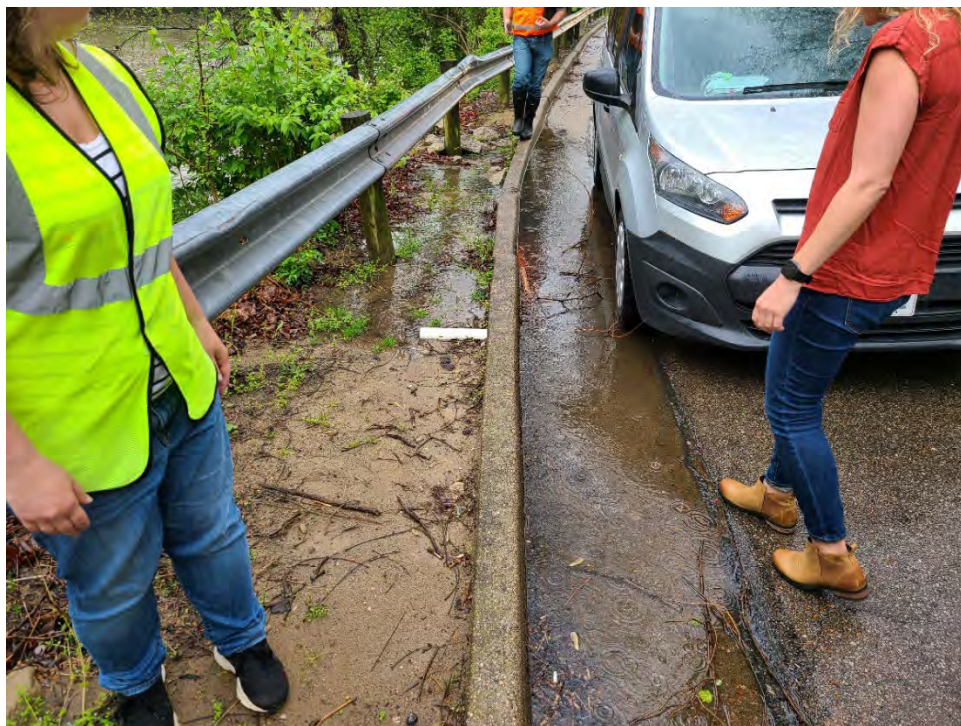
Photo 4 (Site 2): Water ponding on the southeast side of E. Kemper Road (looking southwest). Note inserted PVC drain in curb.
