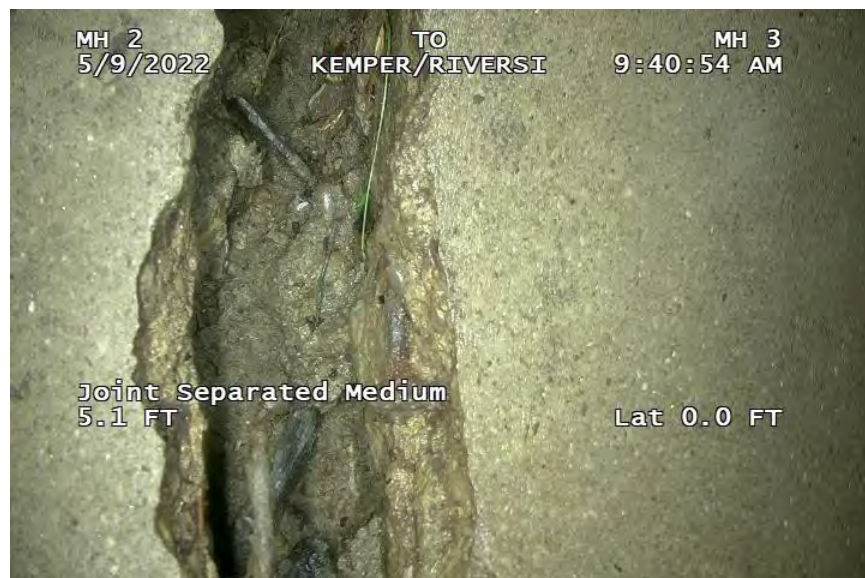
Figure 11: Joint Separation at Site 1
