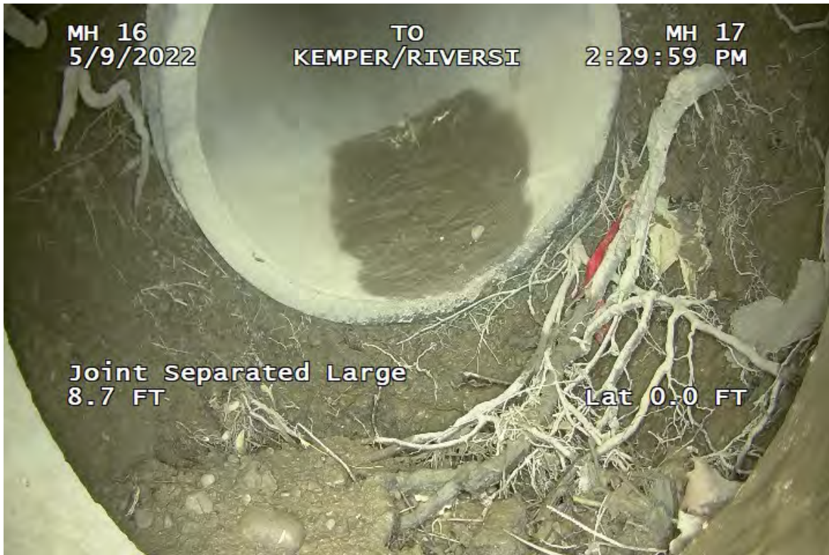
Photo 9 (Site 3): Joint separated at 8.7 feet between MH-16 and HW-17.
