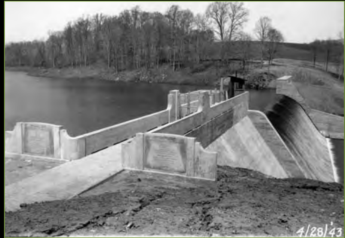
This image from April 28, 1943, shows Atkisson Dam soon after construction was completed in 1942. The U.S. Army Corps of Engineers constructed the dam to provide water supply to Edgewood Arsenal, now known as Aberdeen Proving Ground. (Courtesy Photo)
