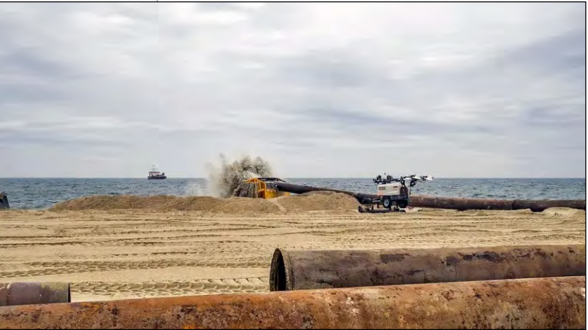
Sand is dredged and pumped onto the Atlantic coast of New Jersey as part of a USACE beach erosion control project. (Photo courtesy of NJ Spotlight)
