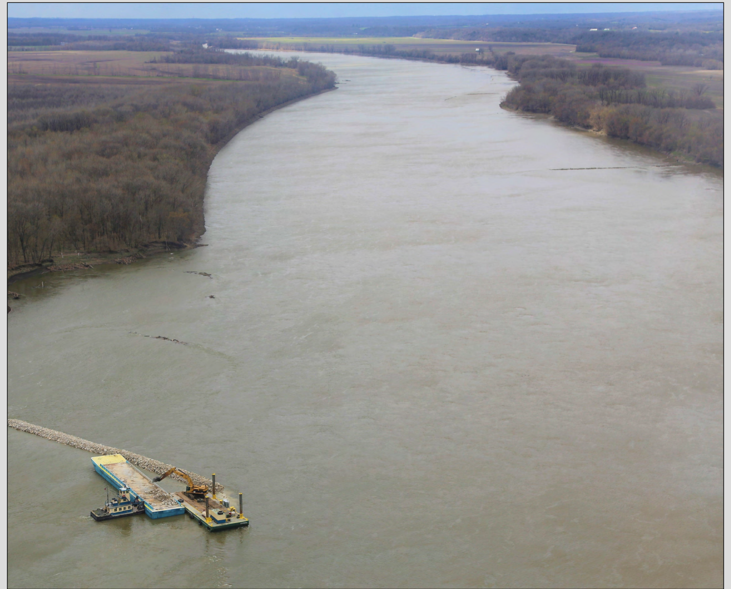
Newt Marine, a contractor, places rock on a damaged river structure on the Missouri River April 7, 2022. Flooding in the region caused an estimated $2.9 billion in damages across the Midwest in 2019. (Photo by Dane Morris)
