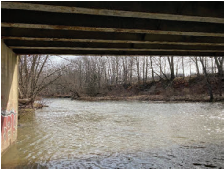
Photo 5: Looking upstream under Griffey Rd bridge
