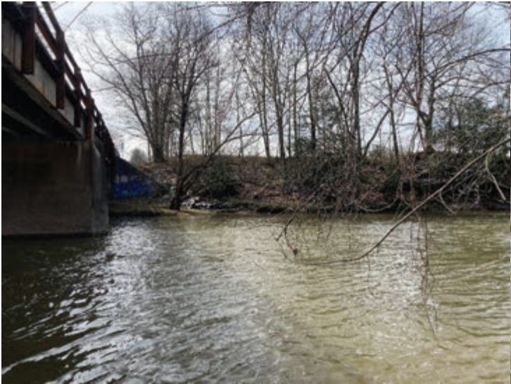
Photo 7: Looking downstream next to Griffey Rd bridge
