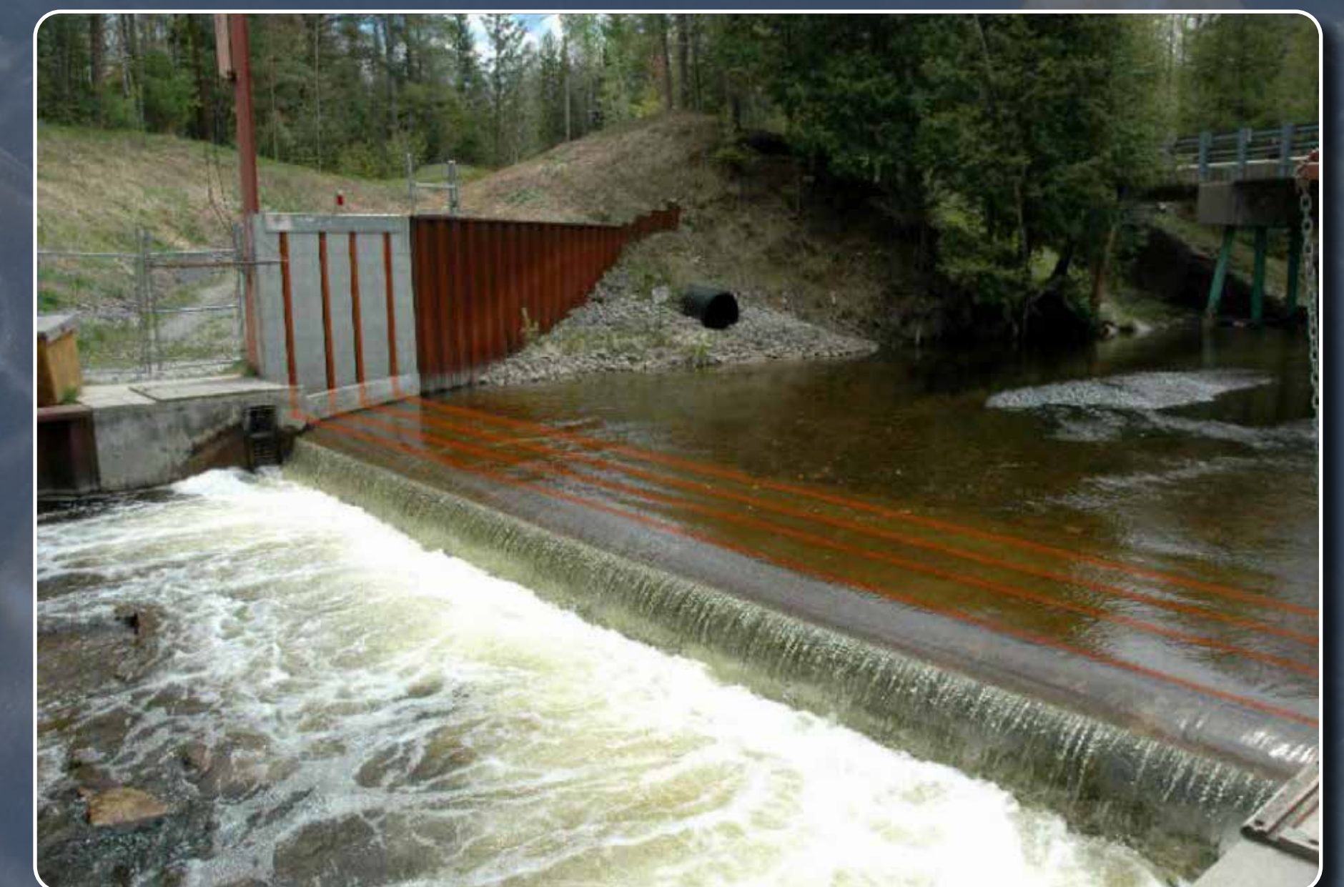
Combined fixed-crest and electric barrier on the Ocqueoc River, Michigan (Source: Zielinski et al, 2019)
