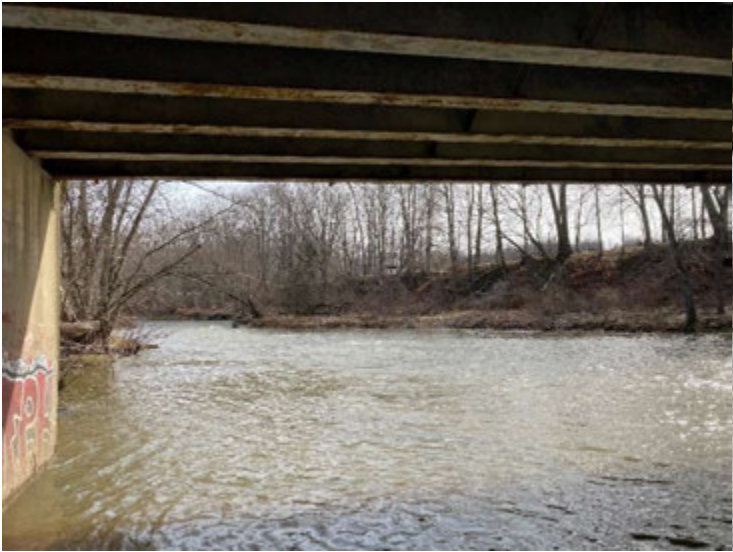
Photo 5: Looking upstream under Griffey Rd bridge
