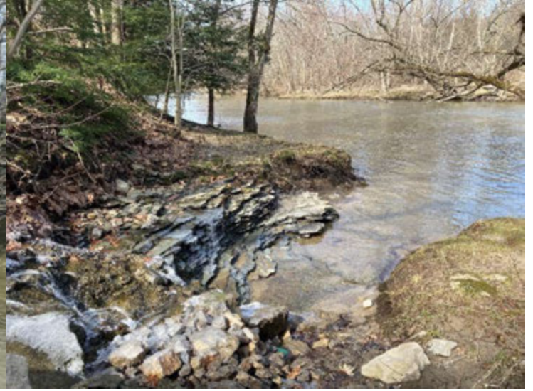
Photo 14: Effluent from culvert near Griffey Rd bridge
