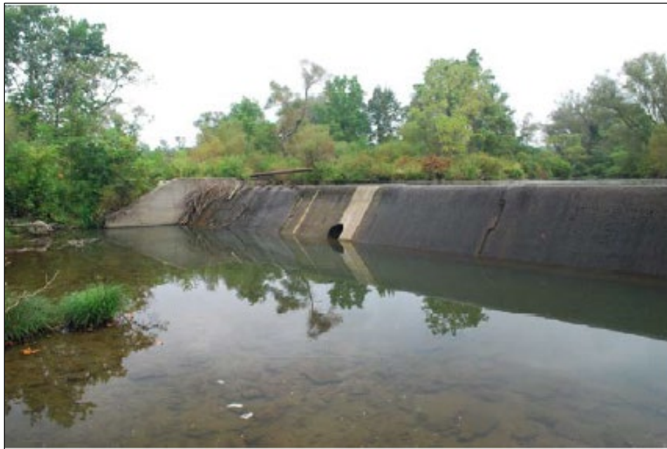
Figure 10: Bessemer Dam on the East Branch of Conneaut Creek, view looking upstream (Photo: USACE).
