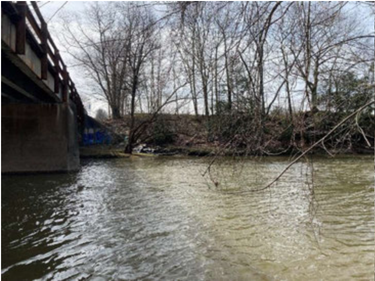
Photo 7: Looking downstream next to Griffey Rd bridge
