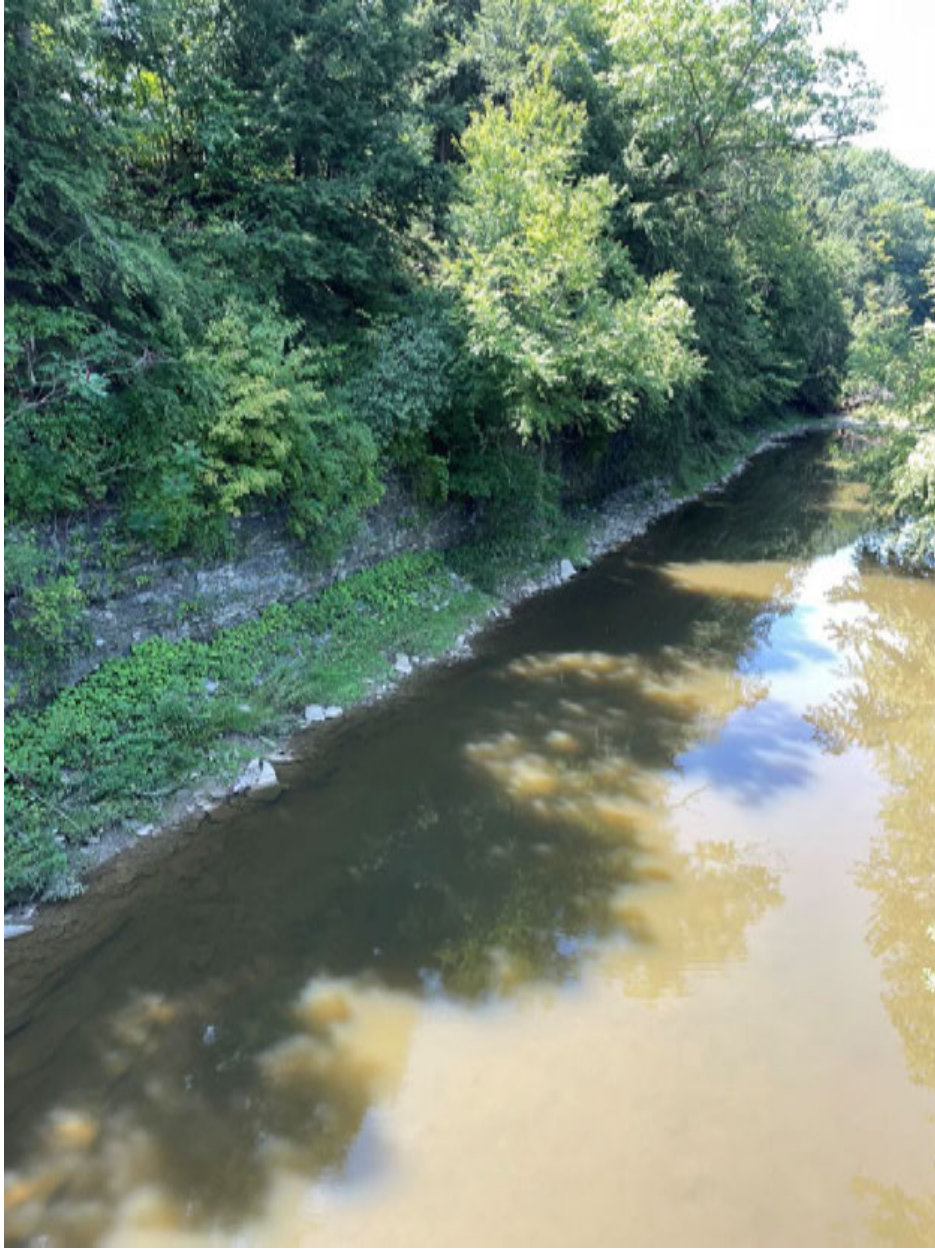
Figure 3. Exposed Shale Bedrock Wall on the Left Bank of Conneaut Creek, Downstream of Route 6N.
