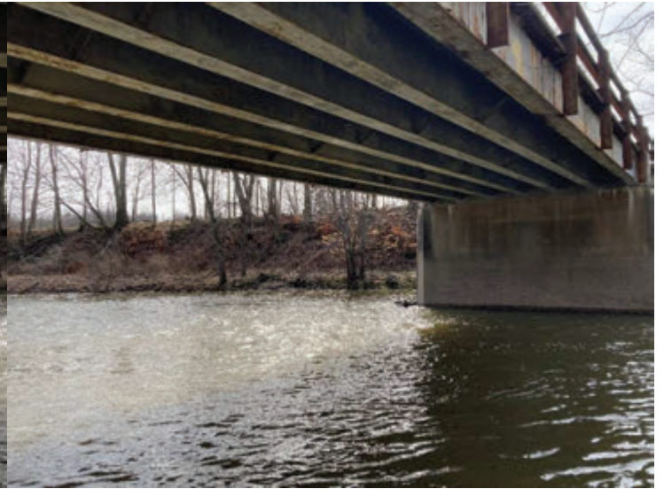
Photo 6: Looking upstream under Griffey Rd bridge
