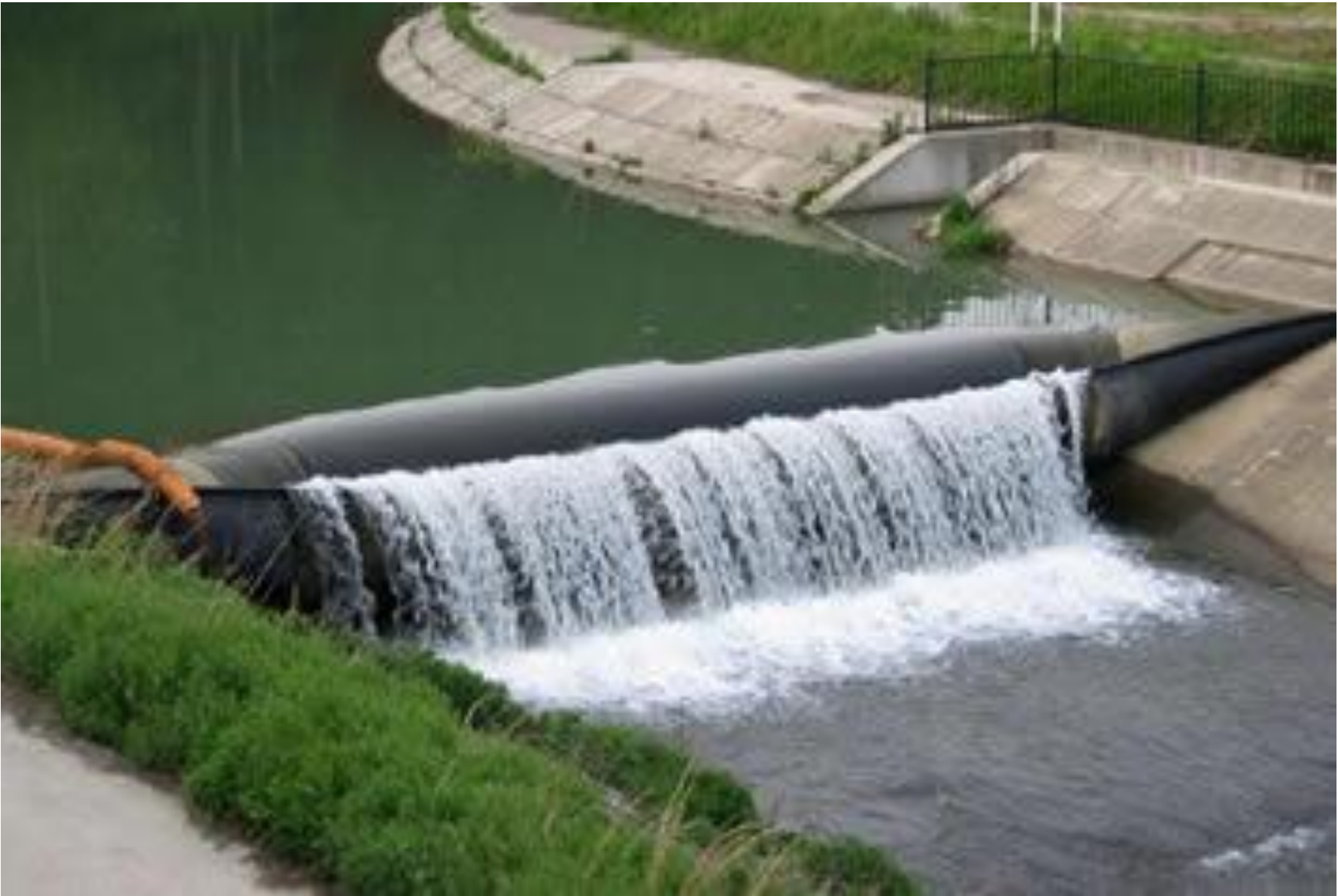
Figure 12: Example of Inflatable Rubber Dam (Source: https://www.rubberdam.org/product/bookend-rubber-dam.html )
