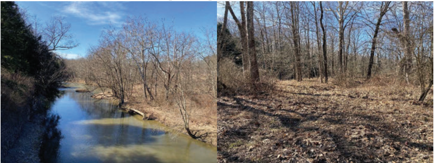
Photo 44: Looking downstream from Route 6N bridge
