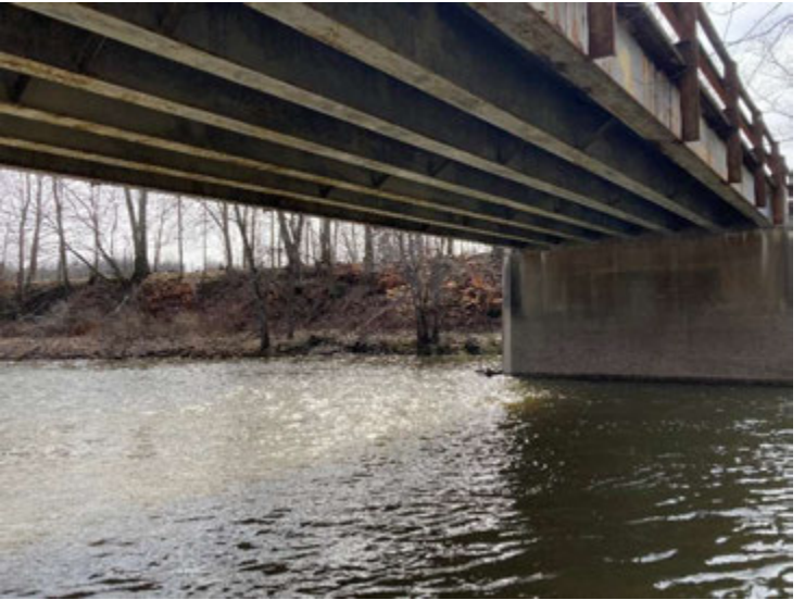
Photo 6: Looking upstream under Griffey Rd bridge
