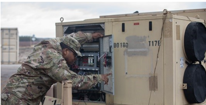
Pfc. Tariq Wrighinton, a utilities equipment repairer, assigned to Headquarters and Headquarters Company, 3rd Division Sustainment Brigade, 3rd Infantry Division, works on a deployable rapid-assembly shelter heater during a convoy live fire exercise in Swietoszow, Poland, Feb. 6. (U.S. Army photo by Spc. Elsi Delgado)
