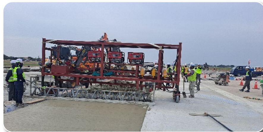
Repair Pavement on Runway, Kunsan Air Base
