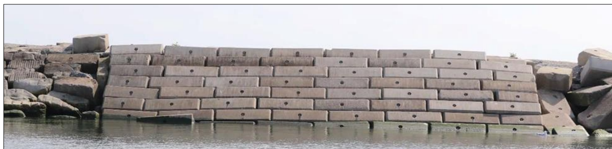
Figure 5: West Breakwater 2012 Repair with Precast Concrete Blocks, June 2016
