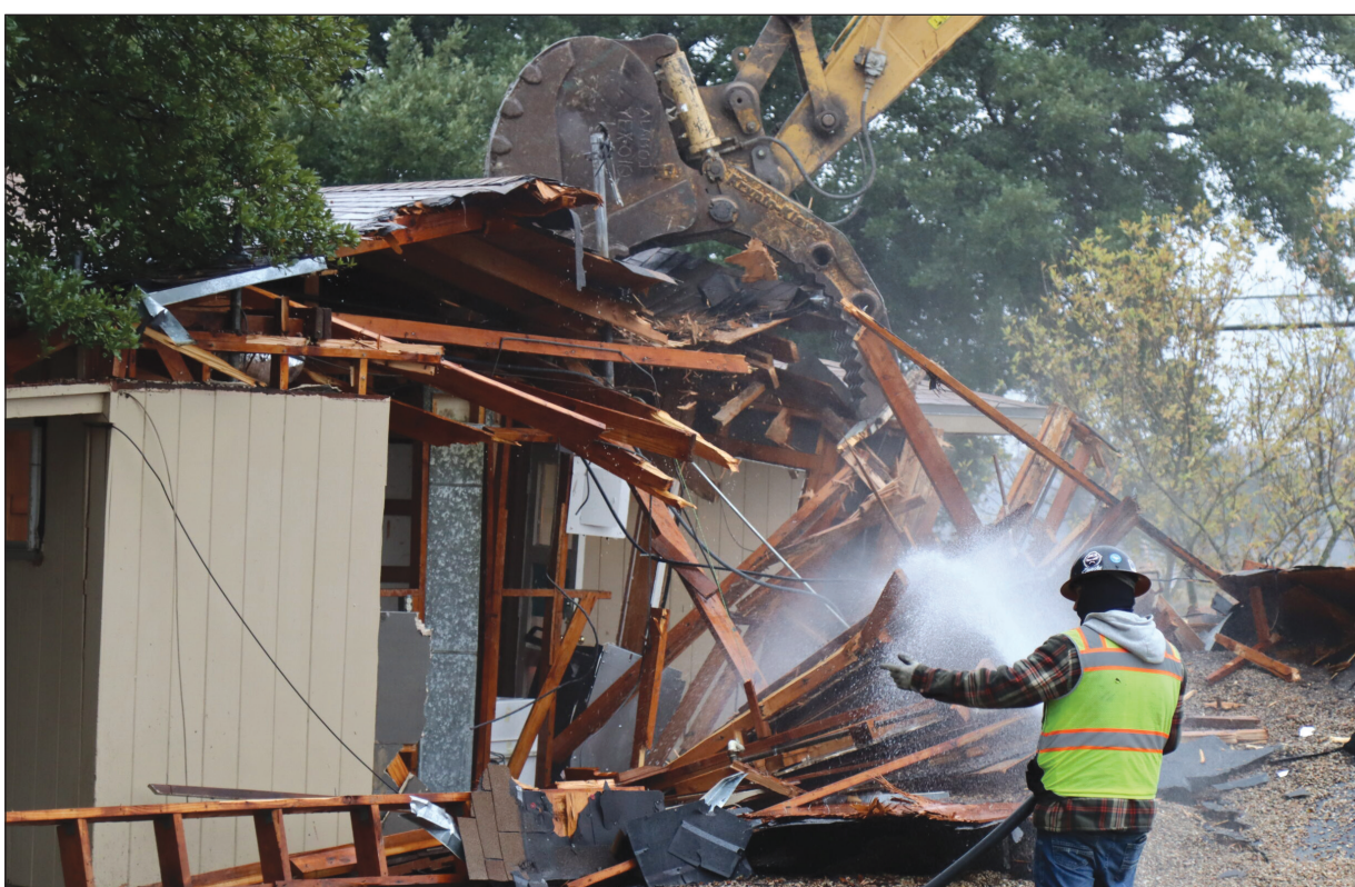
Photo by Shawn Davis, Fort Cavazos Public Affairs A contractor from Lendlease hoses down debris from demolished housing in former Chaffee Village neighborhood to control dust on Fort Cavazos.
