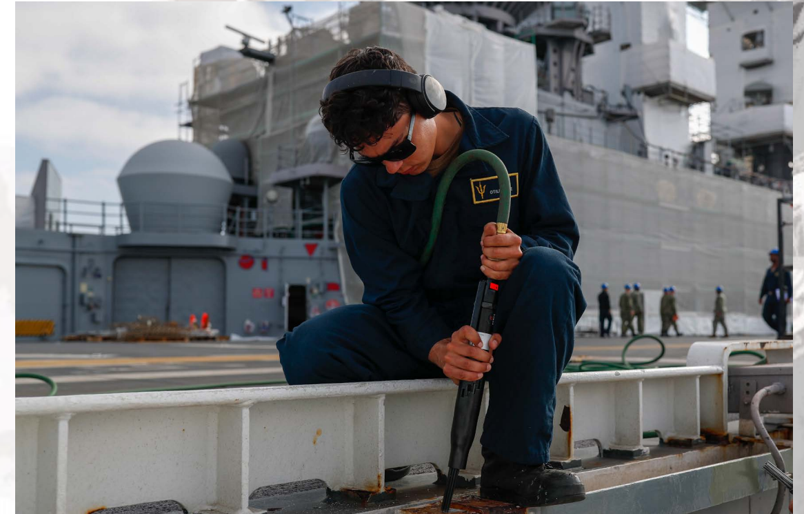
SAN DIEGO (July 5, 2023) -Airman Otilio Diaz, from New York, uses a needle gun to remove paint on the flight deck aboard amphibious assault carrier USS Tripoli (LHA 7) during the ship's maintenance availability July 5. Tripoli is an America-class amphibious assault ship homeported in San Diego. (U.S. Navy photo by Mass Communication Specialist 2nd Class Malcolm Kelley)
