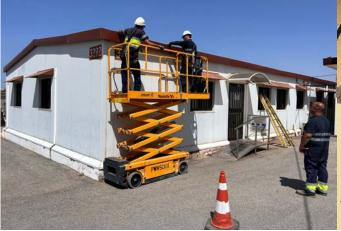
CM3(SCW/EXW) Christopher King is seen above removing an electronic cipher lock that stopped working. Efforts quickly enabled the five Marines to exit from a locked room.
