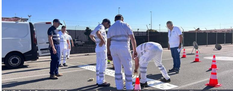
PWD Rota's Facilities & Sustainment Branch personnel are seen here installing a trial speed bumps in front of 158 of PWD Rota complex, under supervision by Rafael Lopez Puyana on July 25th, 2023. After the test bumps pass the tests, more of these are expected to be installed throughout the base, especially around the roundabouts, in order to alert the drivers and mitigate traffic accidents.
