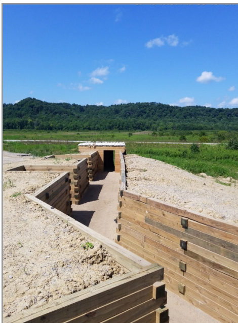
A battlefield trench and machine gun bunker of Fort Knox's digital air-ground integration range are completed and are awaiting revegetation.
