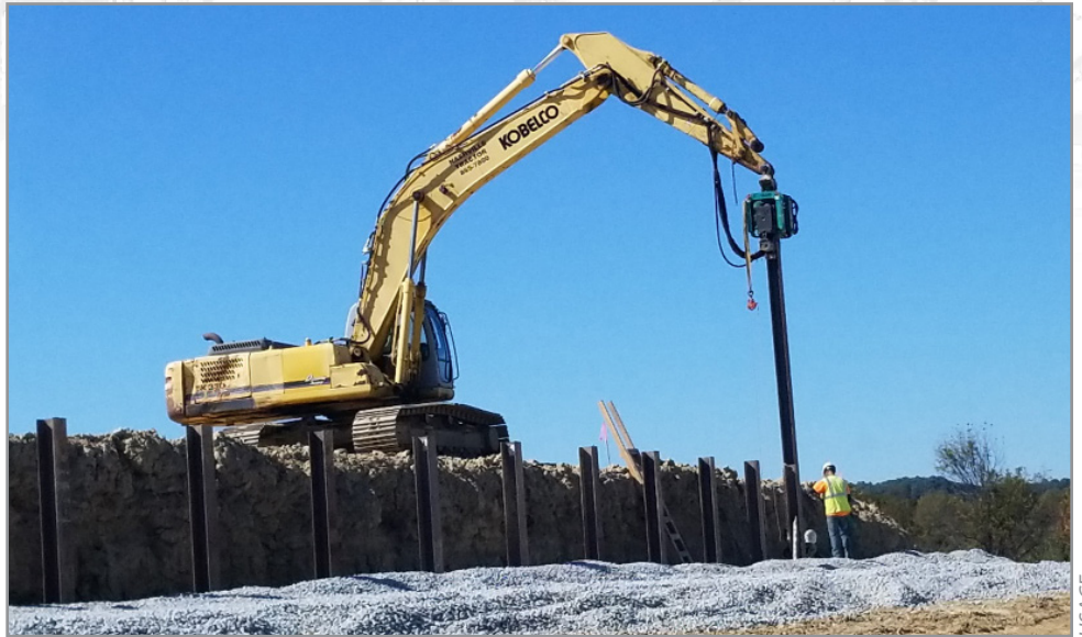
A berm wall of a mobile armor target is being constructed with steel h-piles and wooden railroad ties.
