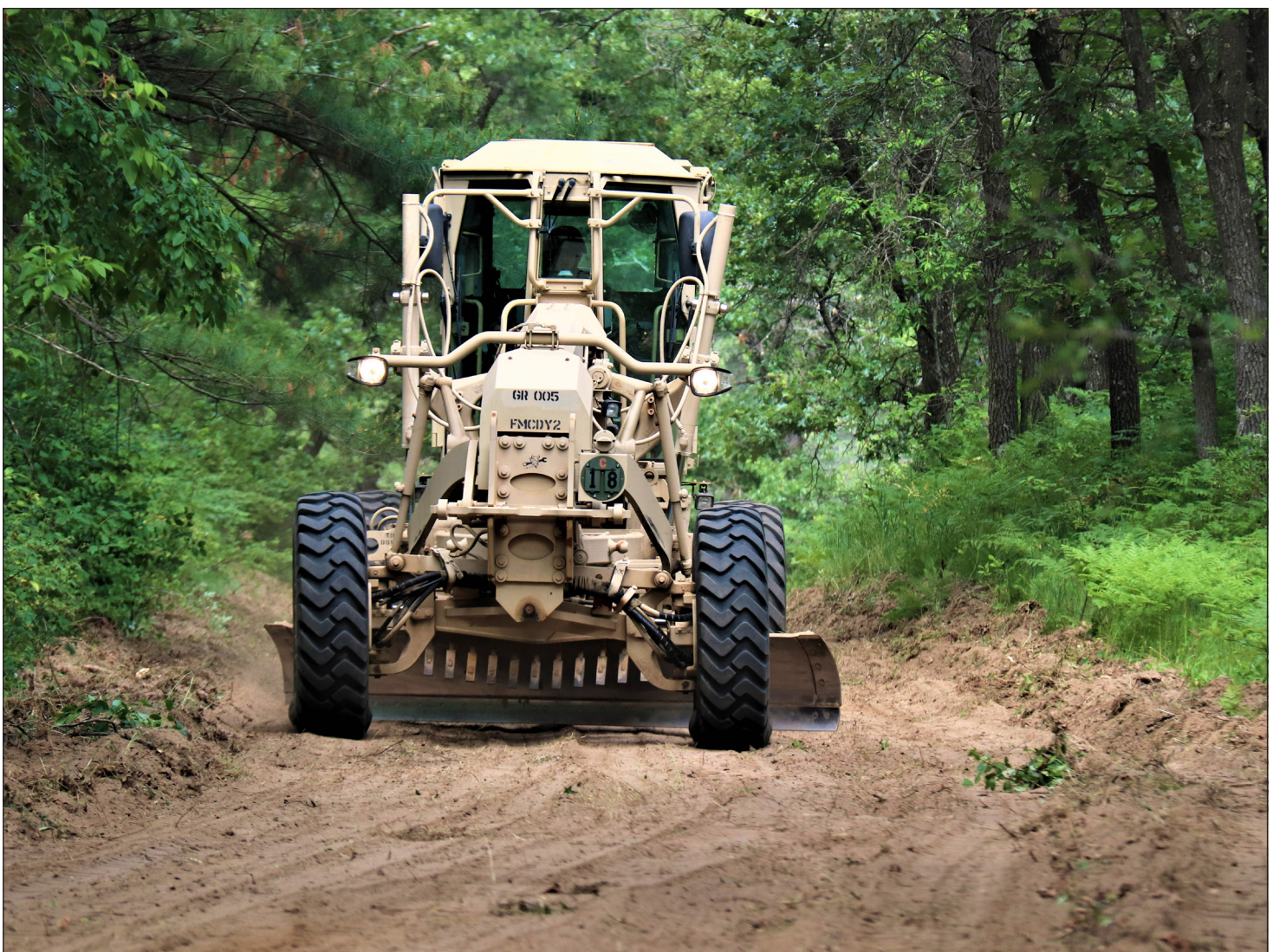
(Above and below) An Army Reserve Soldier with the 411th Engineer Company of the Rear Detachment operates a grader June 12 to re-grade a road on North Post at Fort McCoy as part of a troop project at the installation. The 411th had several Soldiers supporting several troop projects at Fort McCoy in June 2023 to not only get training for those Soldiers but also help Fort McCoy improve its infrastructure.
