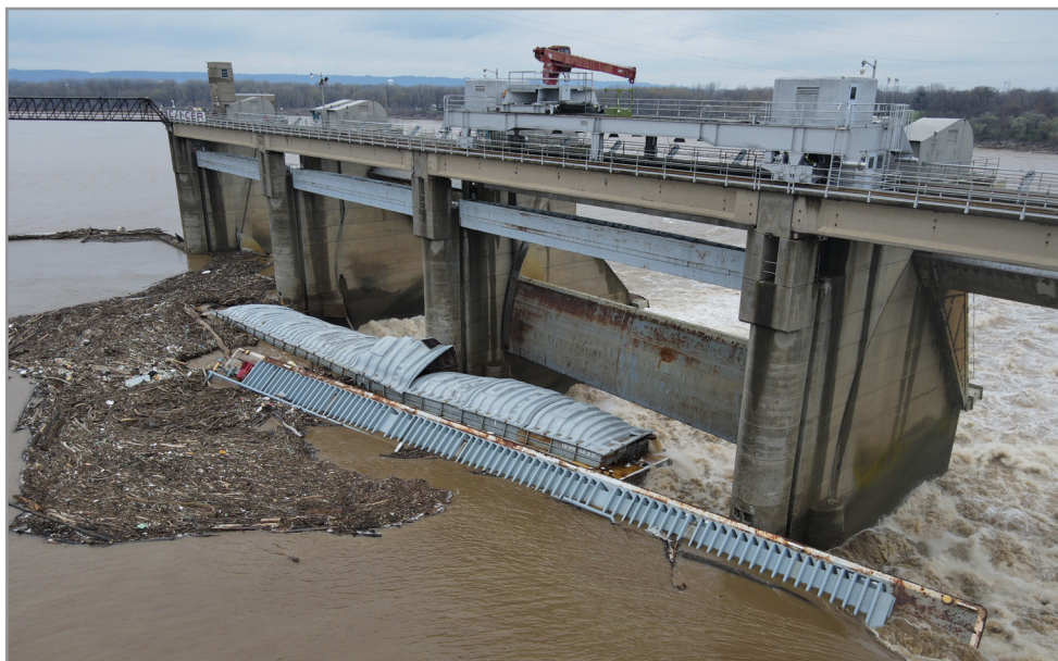
Two barges owned by Ingram Barge Company are pinned against McAlpine Lock and Dam’s lower dam site after the barges broke loose from the towing vessel when approaching the Portland Canal on the Ohio River in Louisville, Kentucky.
