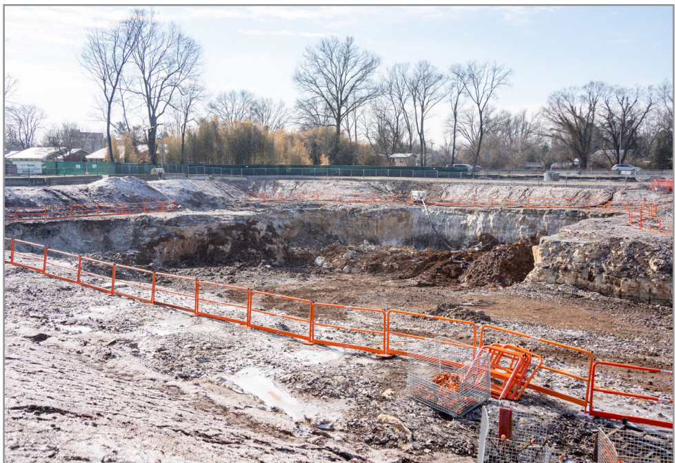
A contractor uses a hoe ram to clear out bedrock in preparation for installing a rainwater storage tank on the site of the new Louisville VA Medical Center Feb. 15, 2023.
