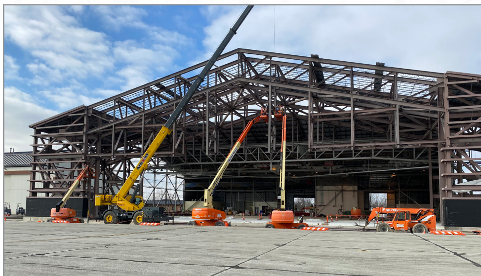
The Grissom Hangar 437 project consisted of an 13,700 square feet expansion and renovation to the existing Nose Dock 5 facility on Grissom Air Reserve Base in Indiana.
