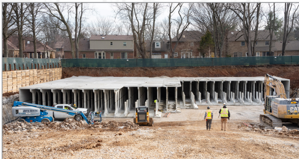
The Louisville District's Veterans Affairs team included the construction of four underground stormwater collection tanks in the plans for the new facility.
